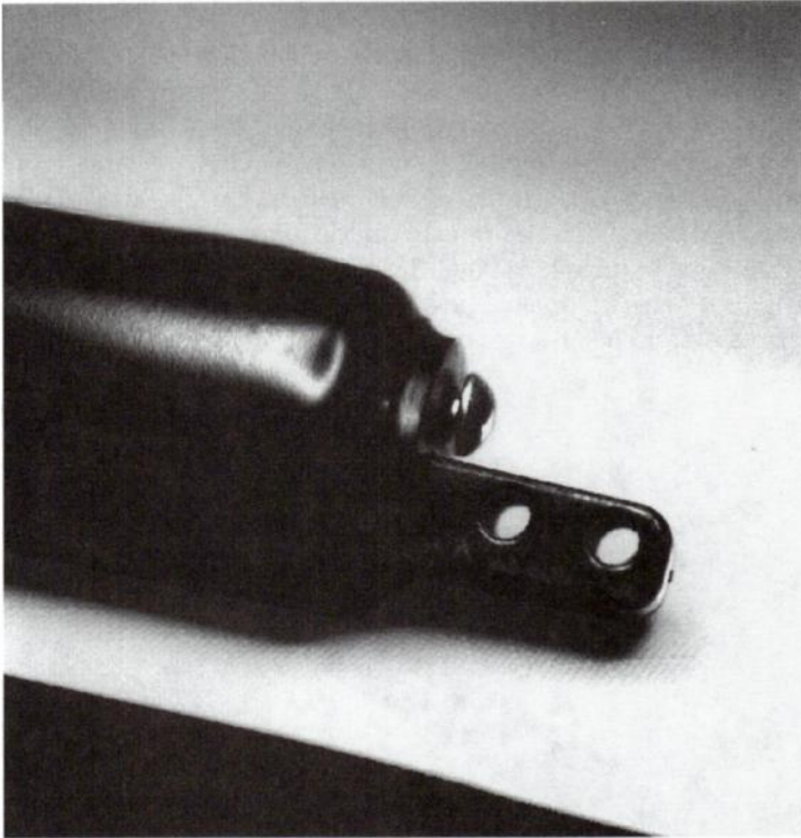
9-10 Closeup of door closer showing position of adjustment screw.
