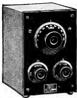
FIG. 137.—Westinghouse single circuit regenerative receiver.
