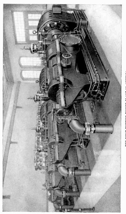
THE FIRST TURBINE POWER PLANT IN AMERICA An Installation of Four 400-Kilowatt Turbine Units at Wilmerting, Penna. This Plant Has Been in Continuous Operation Since August, 1899. Westinghouse Electric & Manufacturing Co., Pittsburg, Penna.
