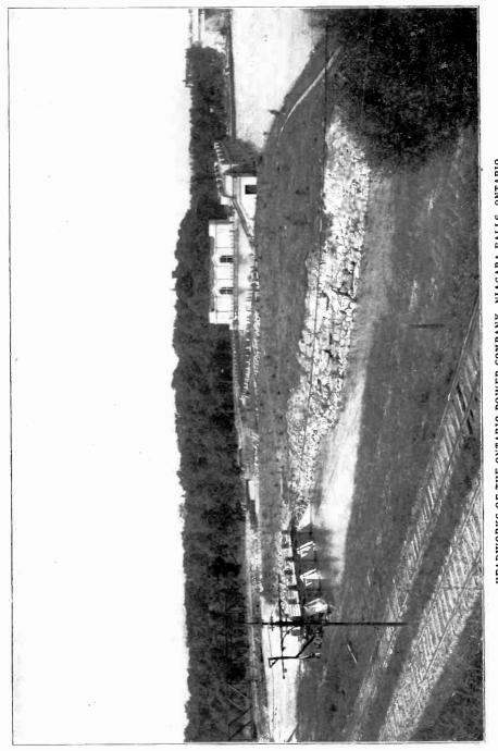
View showing outer and inner forebays, with screen house between. Gate house at further end of inner forebay. HEADWORKS OF THE ONTARIO POWER COMPANY, NIAGARA FALLS, ONTARIO
