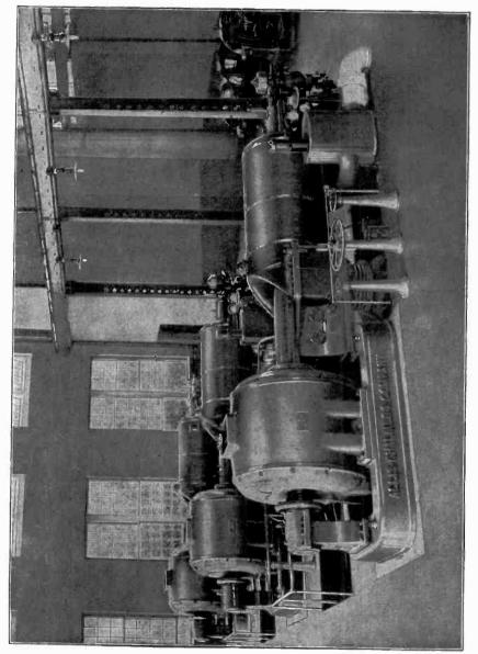
THREE ALLIS-CHALMERS STEAM TURBINES AND GENERATORS 3,250 Kilowatt Installation. Allis-Chalmers Co., Milwaukee, Wis.
