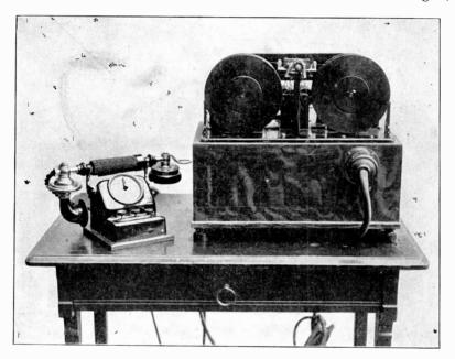
Fig. 5. Wire Type of Telegraphone. Indicator at left.
