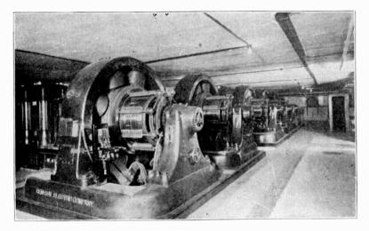
Fig. 21. Rotary Converters in Basement of Office Building.
