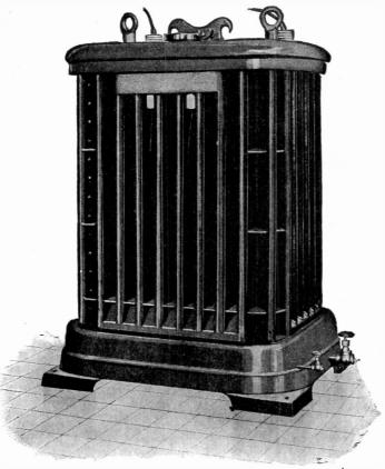
Fig. 15. Oil-Cooled Transformer
