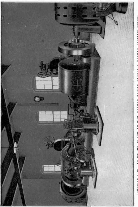
INTERIOR VIEW OF POWER PLANT OF THE DALTON POWER COMPANY, DALTON, MASSACHUSETTS Two units of 21-inch "New American" turbines, operating under 152 feet head.
