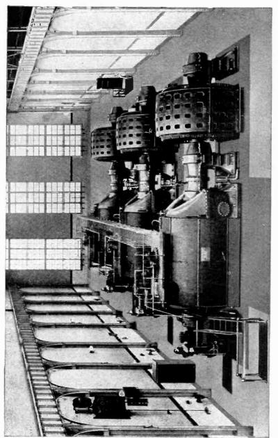
Fig. 89. Three Westinghouse-Parsons Steam Turbines Showing Divided Casing
