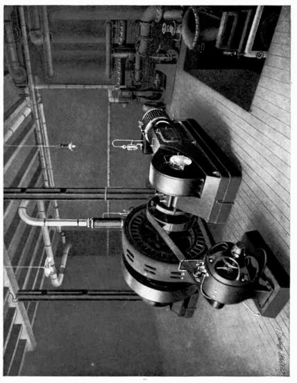
HORIZONTAL CROSS-COMPOUND SINGLE-VALVE ENGINE, DIRECT-CONNECTED TO GENERATOR
