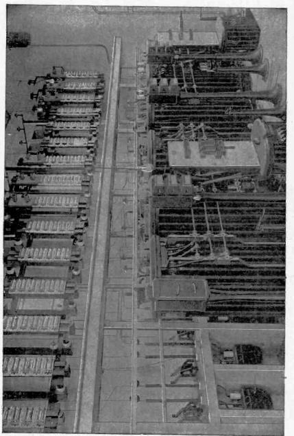
Fig. 35. Typical Installation of Lightning Arresters
