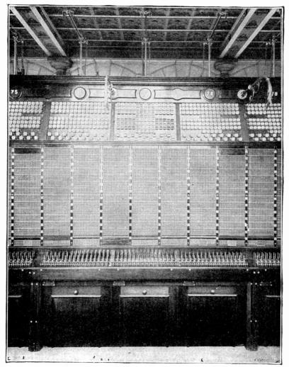
Fig. 181. Face of Magneto Multiple Switchboard
