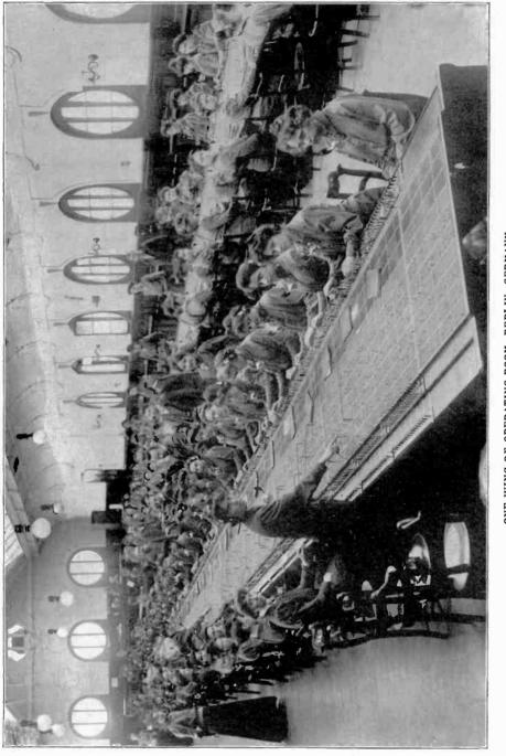
**ONE WING OF OPERATING ROOM, BERLIN, GERMANY** Ultimate Capacity 24,000 Subscribers' Lines and 2,100 Trunk Lines. Siemens-Halske Equipment. Note Horizontal Disposal of Multiple Jack Field.
