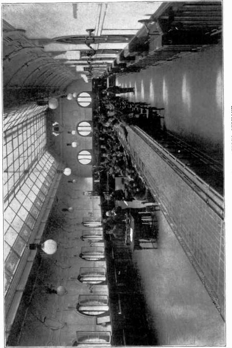
ONE WING OF OPERATING ROOM, BERLIN, GERMANY Ultimate Capacity 24,000 Subscribers' Lines and 2,100 Trunk Lines. Siemens-Halske Equipment. Note Horizontal Disposal of Multiple
