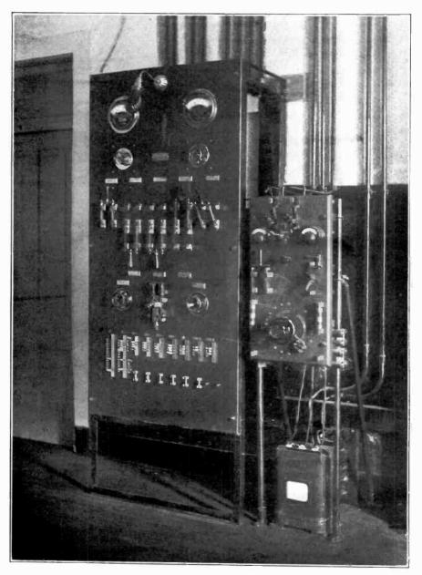
POWER SWITCHBOARD FOR MEDIUM-SIZED CFFICE Mercury Arc Rectifier Panel and Transformer at Right.
