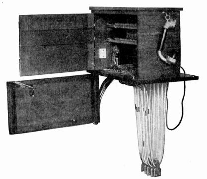
Fig. 152. Sectional Switchboard-Wall Type
