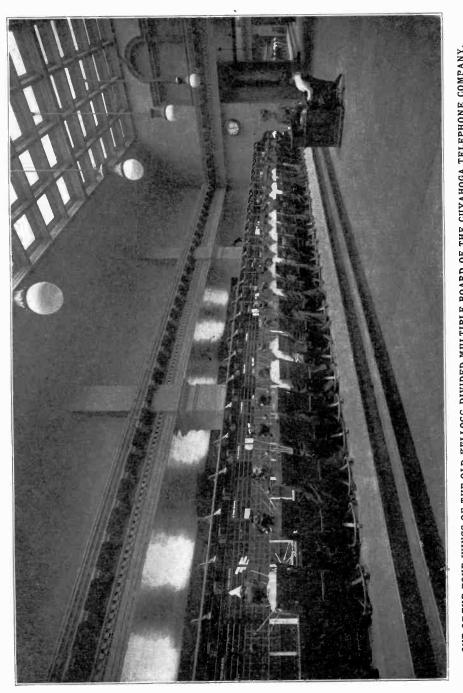
ONE OF THE FOUR WINGS OF THE OLD KELLOGG DIVIDED MULTIPLE BOARD OF THE CUYAHOGA TELEPHONE COMPANY, CLEVELAND, OHIO Ultimate Capacity, 24,000 Lines. One of the Two Examples in the United States of a Multiple Switchboard Having an Ultimate Capacity over 18,000 Lines. Replaced Recently by a Kellogg Strafght Multiple Board Having an Ultimate Capacity of 18,000 Lines and a Present Capacity of 10,000 Lines.
