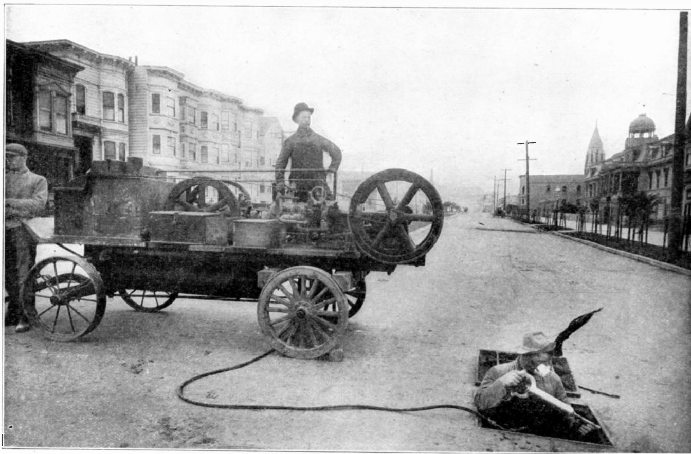
COMPRESSED AIR WAGON FOR PNEUMATIC DRILLING AND CHIPPING IN MANHOLES
