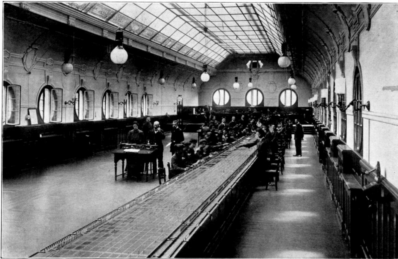
ONE WING OF OPERATING ROOM, BERLIN, GERMANY Ultimate Capacity 24,000 Subscribers' Lines and 2,100 Trunk Lines. Siemens-Halske Equipment. Note Horizontal Disposal of Multiple
