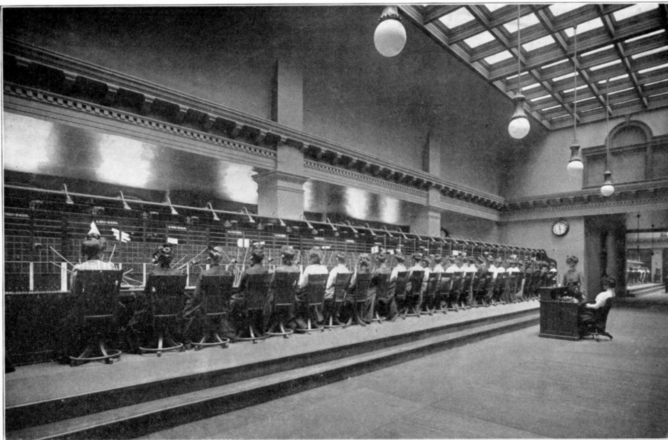
ONE OF THE FOUR WINGS OF THE OLD KELLOGG DIVIDED MULTIPLE BOARD OF THE CUYAHOGA TELEPHONE COMPANY, CLEVELAND, OHIO
