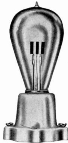
Fig. 212. Vacuum Arrester
