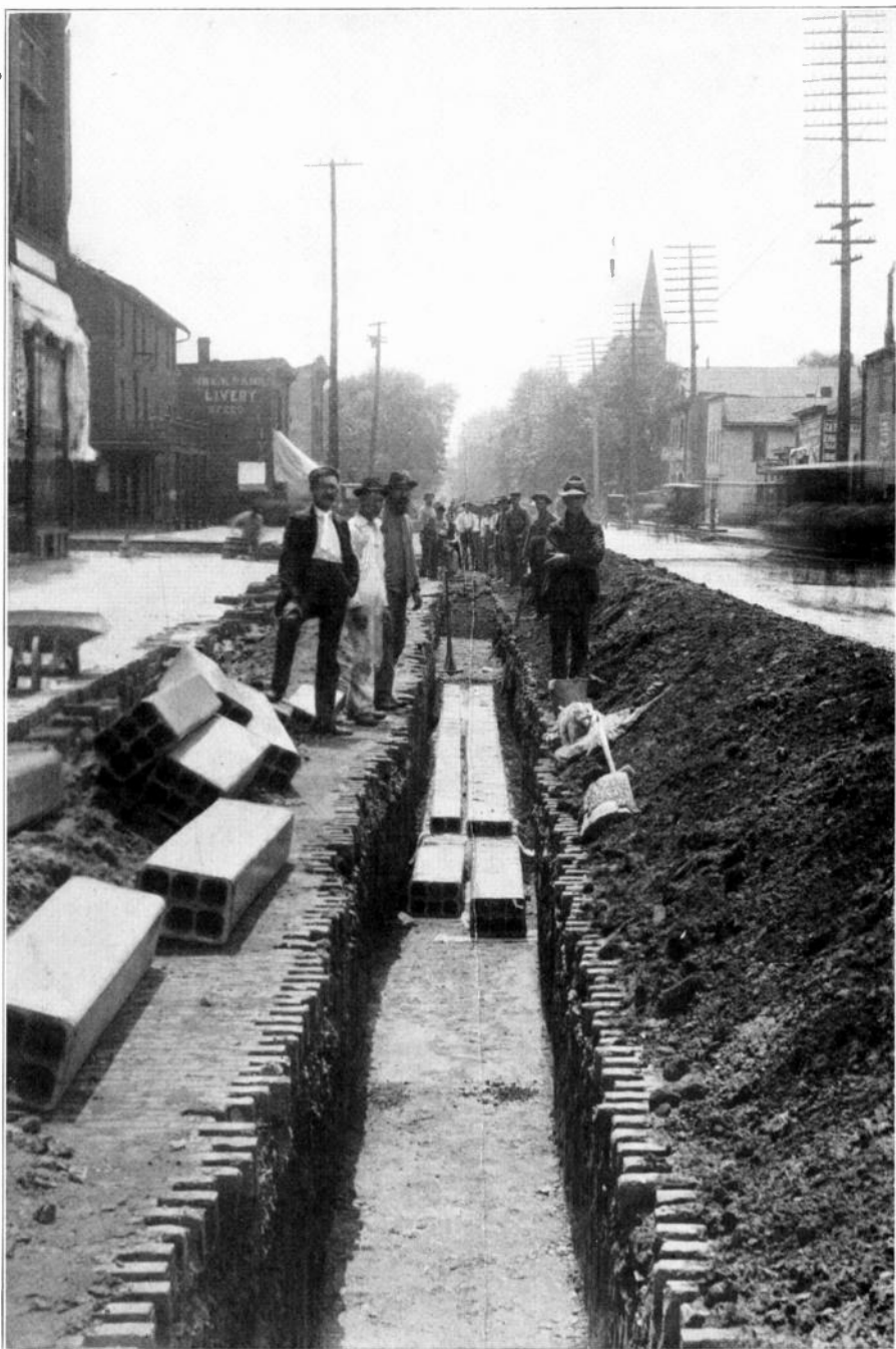
INSTALLATION OF TELEPHONE CONDUIT EMPLOYING MULTIPLE-DUCT TILE Note the Wrapping for Joints.
