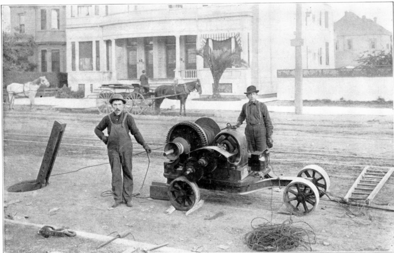
ELECTRIC WINCH FOR DRAWING CABLES INTO UNDERGROUND DUCTS
