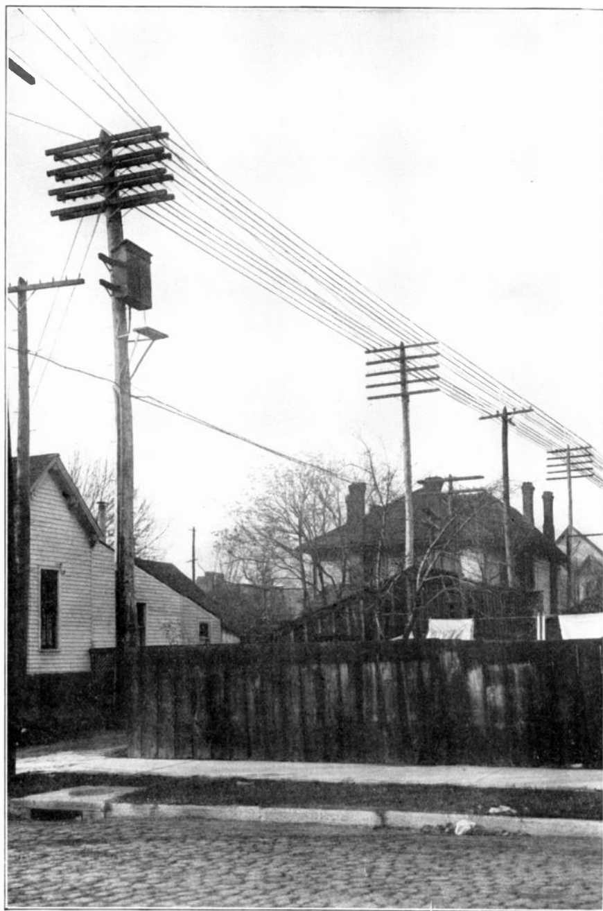
AN UNDERGROUND CABLE TERMINAL FEEDING TO AERIAL
