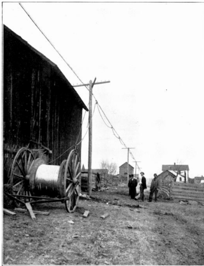
ERECTING SMALL AERIAL CABLE USING MATTHEWS CABLE TROLLEY Scenes at Beginning and End of Run.
