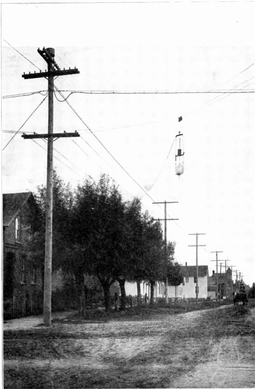
JOINT AERIAL CONSTRUCTION Telephone and Electric Light Wires.
