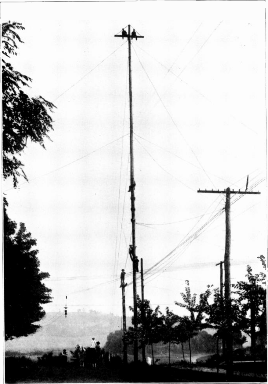
TERMINAL POLE FOR LONG SPACE ACROSS OHIO RIVER AT GALLIPOLIS, OHIO A Better Practice is to Use Steel Towers.
