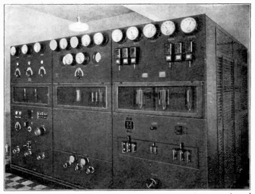
FIG. 34.—The main unit of the 1005-A 5-kw. broadcast transmitter equipment manufactured by the RCA.
