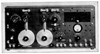
F1G. 67.-Commercial long-short wave receiver, type IP-501A, containing detector and audio-amplifier system.
