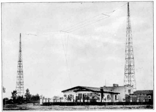
FIG. 81.-Illustrating "T" type antenna and supporting towers.
