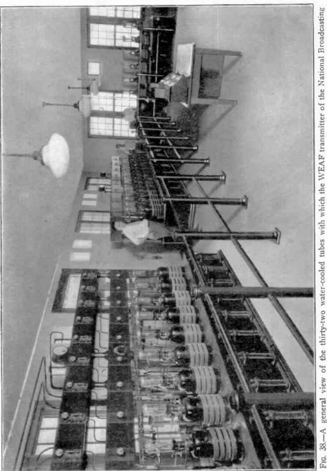
FIG. 38.--A general view of the thirty-two water-cooled tubes with which the WEAF transmitter of the National Broadcasting Company is equipped. Pure water from cooling tanks circulates through the coils of rubber hose at the base of the tubes. Each tube is equipped with a relay which drops and displays a small white disk in case of tube trouble.
