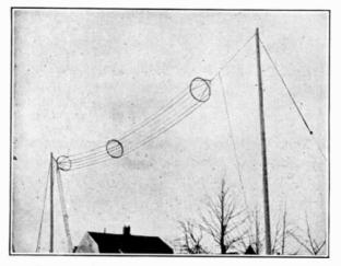
FIG. 44.-Cage type antenna with cage lead-in.
