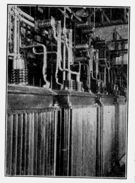
Fig. 322—Bank of High Voltage Transformers at Kahuku.
