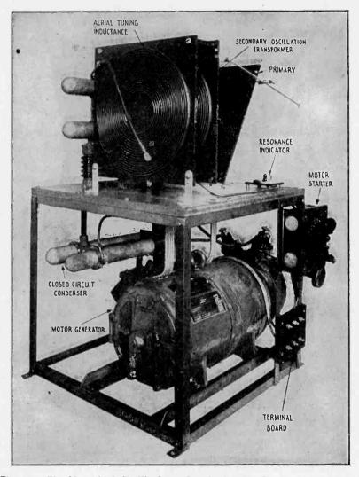
Fig. 266c—The Marconi ¼ K. W. Cargo Set showing the General Arrangement of the Apparatus.
