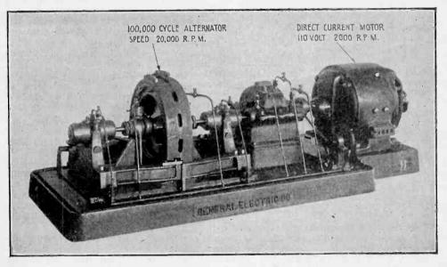
Fig. 280a-The 2 K. W. 100,000 Cycle Alexanderson Alternator.
