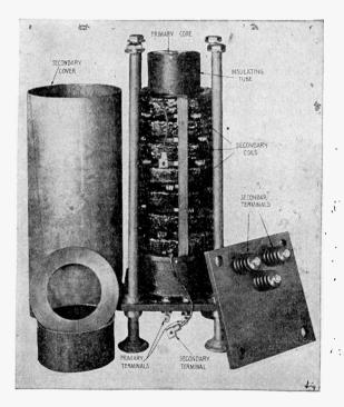
Fig. 131-2 K. W. 500 Cycle Open Core Transformer.
