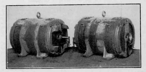
Fig. 67b-2 K. W. Crocker:Wheeler Motor Generator Assembled.
