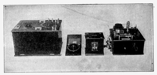
Fig. 277a-The Direction Finder Complete with Fleming Oscillation Valve.
