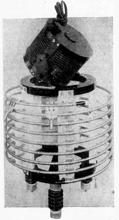
Fig. 119—Type A Oscillation Transformer of the American Marconi Company.
