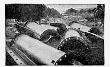
311-Showing Steel Semi-Cylinders for the Marconi Tubular Mast. Fig.
