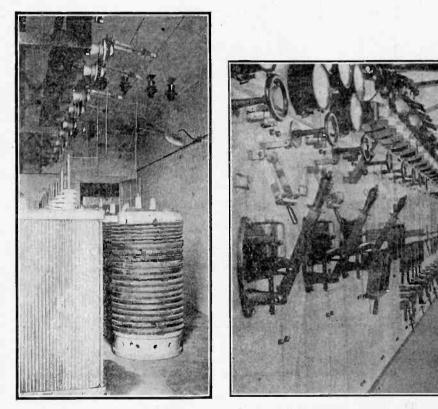
Fig. 307-Bank of High Voltage Transformers at Carnarvon Station.
