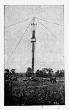
Fig. 313—A Tubular Mast in Early Stages of Construction.
