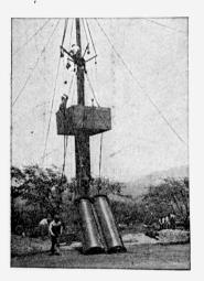
Fig. 312-Showing Workmen's Cage Which is Carried to the Top During the Process of Erection.
