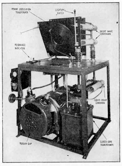
Fig. 266b-The Marconi ¼ K. W. Cargo Type Transmitting Set Complete.
