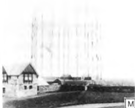
Massive array of antennae at Pol-du, Cornwall, England, to conquer Atlantic. Erected 1901 summer. (Similar to ones erected in Cape Cod, U.S.A.)
