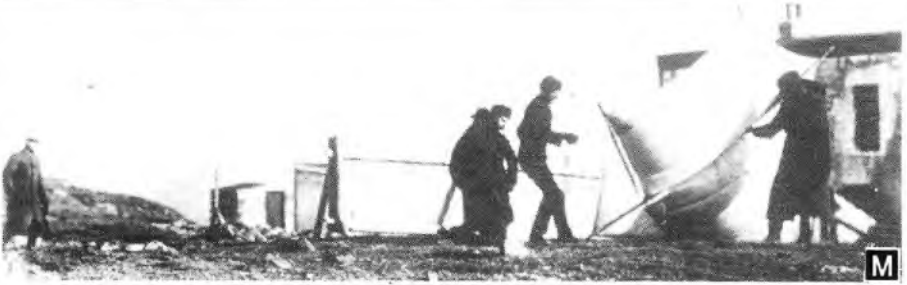
Raising the kite at Signal Hill (apt name!) St. Johns Newfoundland weather too bad for balloons; masts already blown down. It will haul 400 feet of wire aloft and (hopefully) receive signals sent from Poldhu... Marconi on extreme left.
