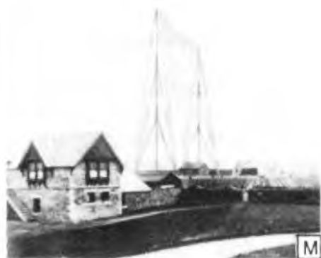
Replacement by two masts only. From here signals sent — letter S— and received in Newfoundland 12 Dec. 1901; there balloon tried, but frequently blown away; so kite used successfully to receive signal.
