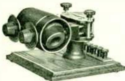
**Broadcast Variocoupler**—Some sets are not designed to tune-in the broadcast entertainments. For these outfits a device such as the one at the left is added to the set for this purpose. It consists of a tube with a rotating coil at each end
