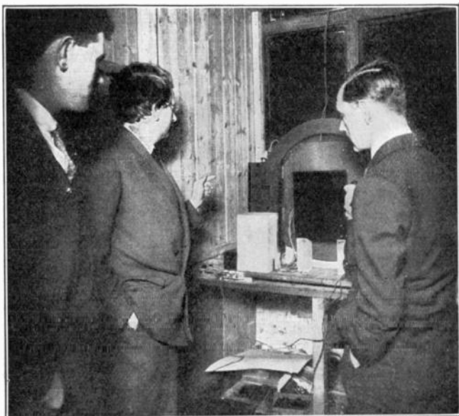
FIG. 85.—A part of the color television apparatus used by J. L. Baird.
