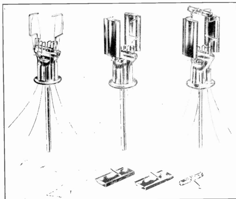
—IN THE MANUFACTURE OF A FULL-WAVE RECTIFIER
