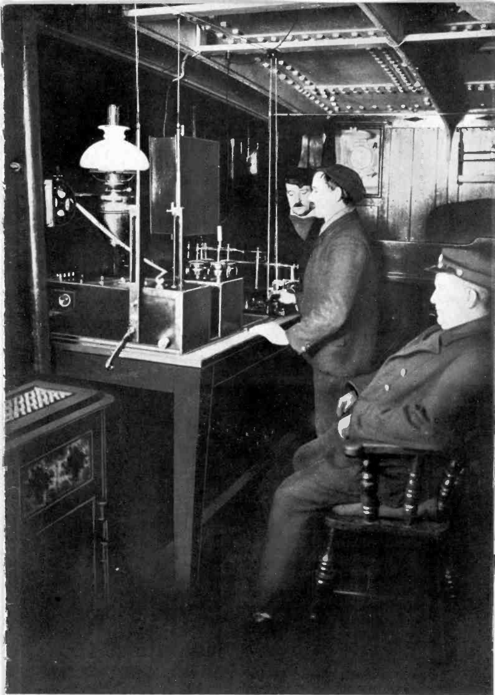
Early Marconi wireless installation on board a lightship, 1898
