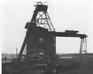
Fig. 2. Shaft House for a deep mine in the Lake Superior region with skip car about to dump and with loaded railway car under the pockets
