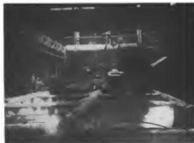
Fig. 16. Concrete tank for granulating cinder with clam-shell grab bucket operated from overhead traveling crane
