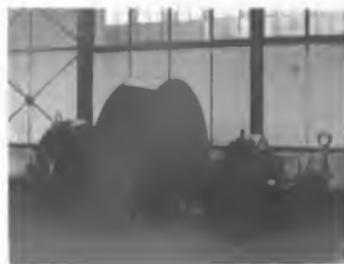
Fig. 14 44 Ton Fly-wheel, Pit Zollern II
