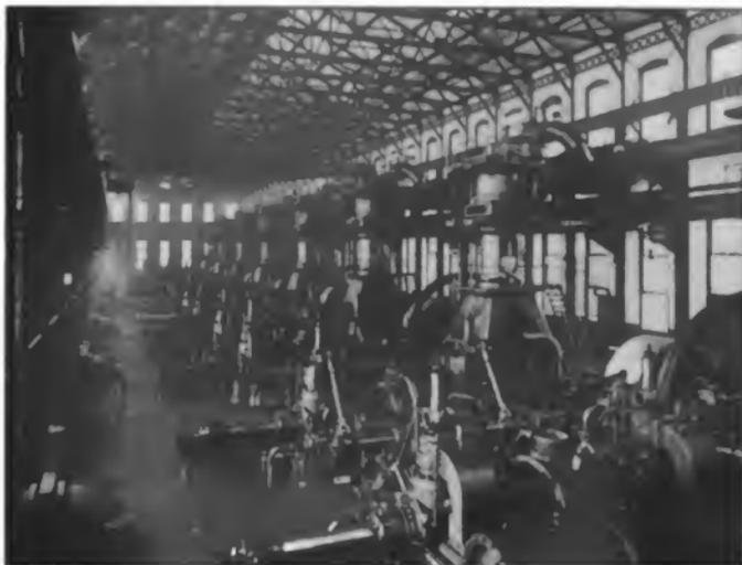
16-2000 Kw. Gas Engines in the Power Plant of the Lackawanna Steel Co.
