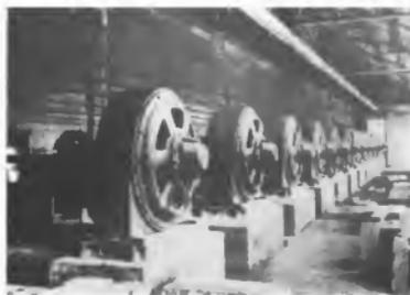
Fig. 4. 124-18-100-160 2 3-K-440 volt motors driving raw material tube mills in Universal Portland Cement Co., Plant No. 4. These motors are coupled through flexible couplings to the countershafts of the mills. This necessitates only one gear reduction. The concrete wall separating the motors from the mills secures an unusually clean motor room.
