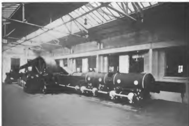
500 H. P. Gas Engine Built by the Sargent Engine Co., Driving
