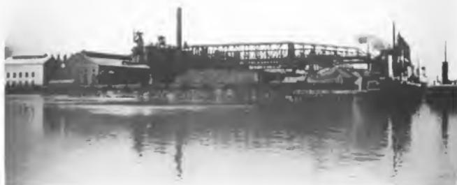
Fig. 17. General view of North Slip, Illinois Steel Company, South Chicago Illinois, showing steamers, ore unloaders, ore bridges and transfer cars and furnaces in the background
