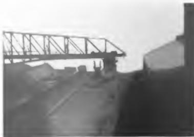
Fig. 4. Ore Bridge with Clam-Shell Grab Discharging Ore into a Transfer Car
