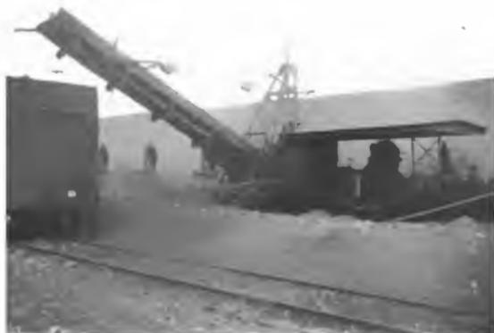
Fig. 2. Rear View of Covington Coke Extractor, Showing Controller for Ram, and Handwheel for Varying Angular Position of Ram Travel
