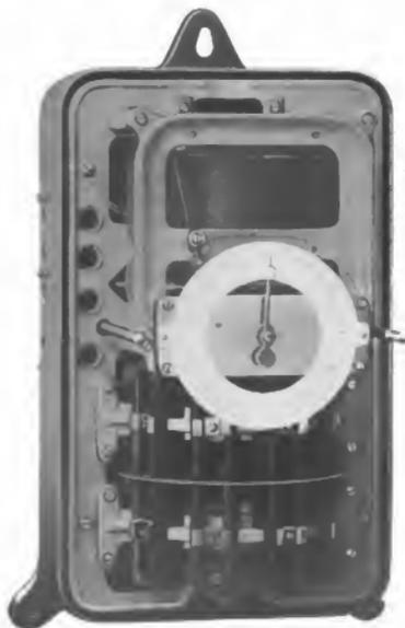
Fig. 2. Maximum Demand Indicator. Cover Removed
