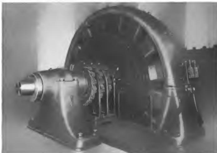
Fig. 1. 16 Pole, 2000 Kw., 188 R.P.M., 600 Volt Six-Phase Rotary Converter
