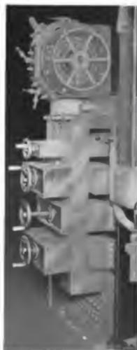
Fig. 4. Switch on Positive Side of 2000 kw. Converter. Sub-station, New York Edison System
