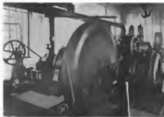
Fig. 10. 125 h.p. Flywheel Motor Generator Set at "Donnersmarkhütte"
