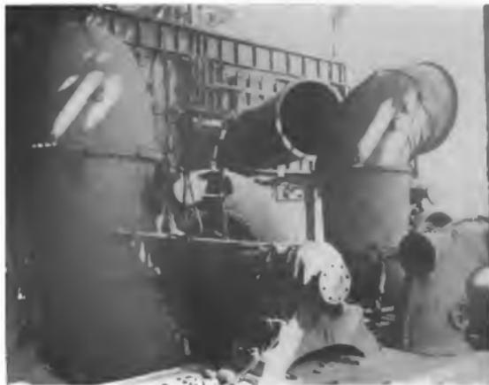
Fig. 7. Installing Water Wheels in Station No. 3
