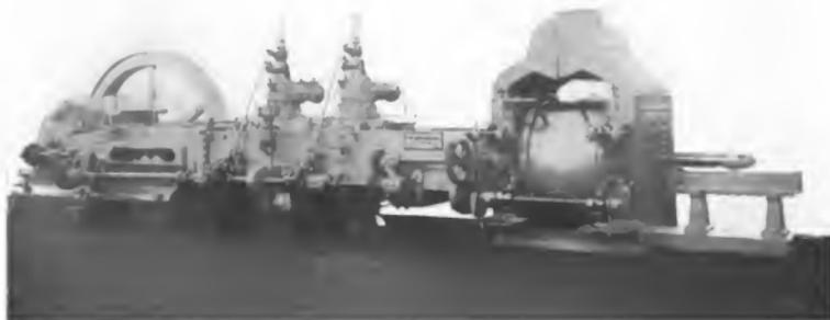
Later Type of Blowing Gas Engine as Built by The John Cockerill Works, Seraing, Belgium
