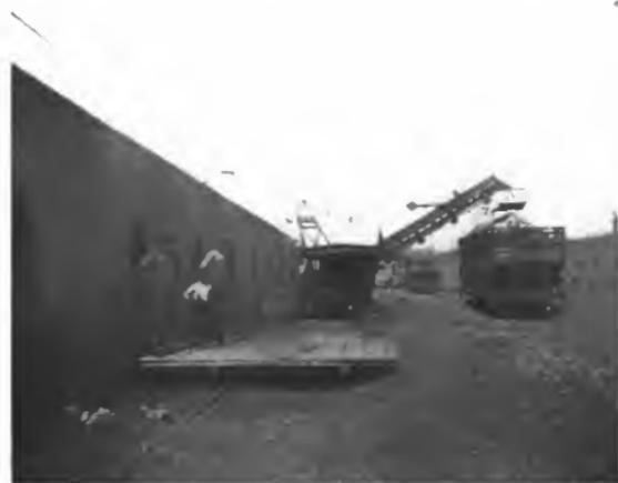
Fig. 1. Covington Coke Extractor drawing Coke from "Beehive" Oven and loading into Car. This Illustration shows arrangement of Ovens at Typical Machine Plant
