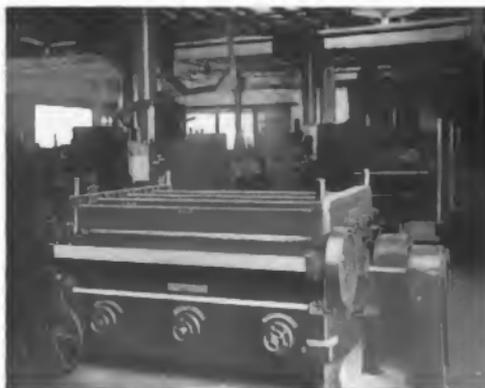
**60" Triple Drum Power Feed Sander Driven by 25 h. p. Motor
