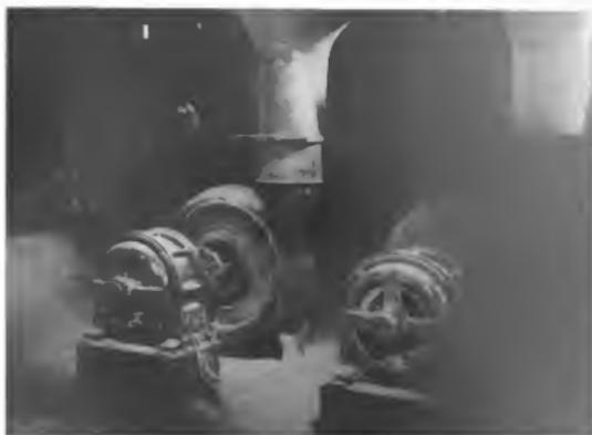
Fig. 1. 2-I-4-10-750-K-440 volt motors flexibly coupled to Buffalo blowers, used to force a mixture of air and coal dust into the slag and limestone dryers. Similar blowers are used for forcing powdered coal into the rotary kilns. The apparent fog around the right hand machine is due to the large amount of dust in the air
