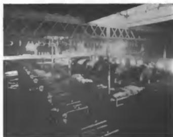
Fig. 7. Filling and Corking Machines. Daily Capacity 250,000 Bottles
