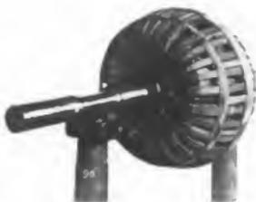
Fig. 4. Armature of Thomson-Houston Dynamo for Incandescent Lighting
