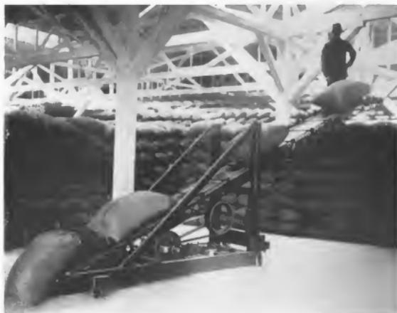
Fig. 1. Brown Portable Elevator Stacking Rough Rice in Sacks
