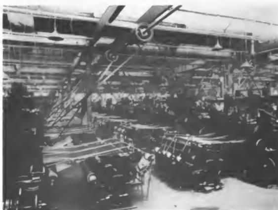
Fig. 2. Weaving Shed, Driven by Line Shafting and Belting, Showing Complication of Belts
