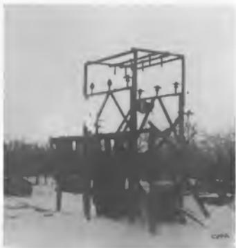
Fig. 1 Fuses Opening Short Circuit on 60,000 Volt System
