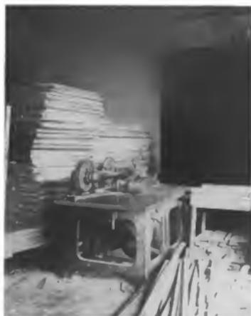
Fig. 3. Automatic Rip Saw Driven by 15 h.p. Constant Speed Motor Located In Basement
