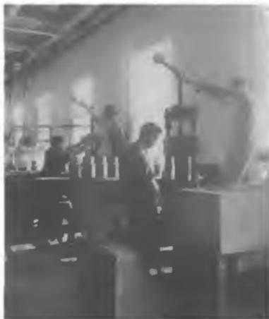
Fig. 4. Presses for Dry-Process Porcelains
