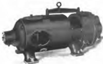
Fig. 3. Type C 20 kw, 125 Volt Non-Condensing Curtis Turbine
