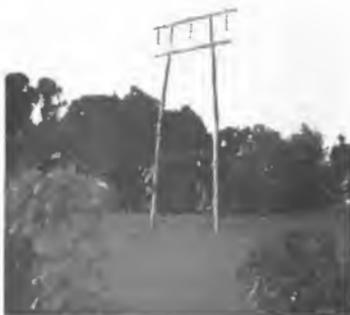
Fig. 7. Transmission Tower equipped with Link Suspension Insulators representing a 125000 volt installation
