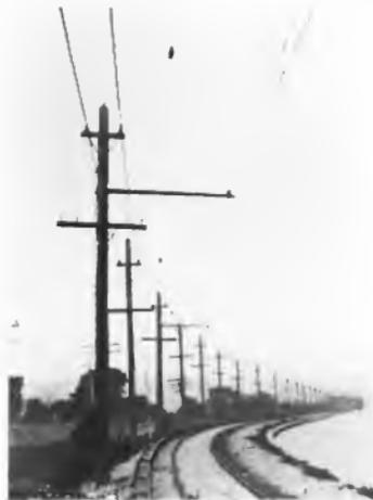
Fig. 5. Strain Insulator as a pull-off installed on a curve on a 6600 Volt Catenary construction
