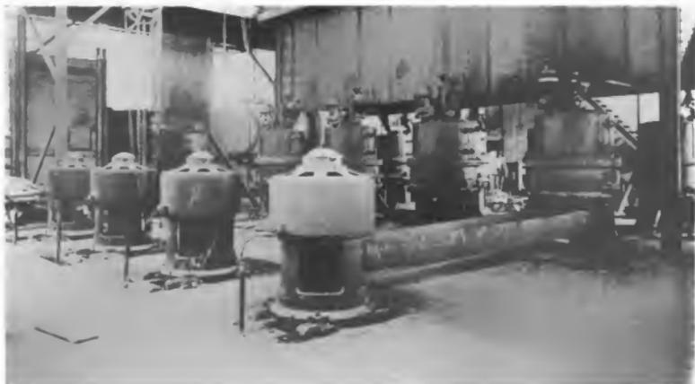
Fig. 5. 1-6-40-500-K-440 volt vertical motors, belted to Fuller mills, Plant No. 4, Universal Portland Cement Co. There are eight of these driven altogether. The bearings on these motors have given entire satisfaction in spite of the dust and grit that naturally tend to produce excessive wear
