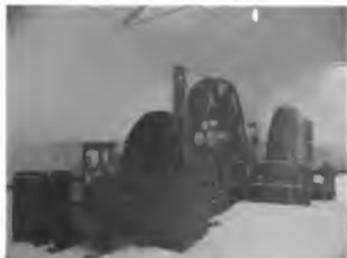
Fig. 23. Hoisting Engine at Pit de Wendel
