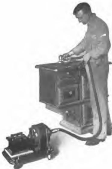
Fig. 1. Stove Polishing Apparatus Driven by 1 2 h.p. Single-Phase General Electric Motor
