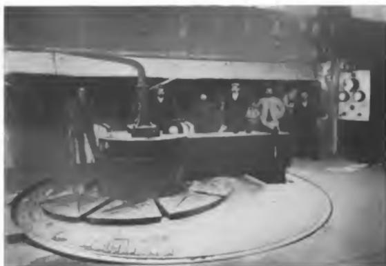
Fig. 6. 450 Kw. Induction Furnace, Top View
