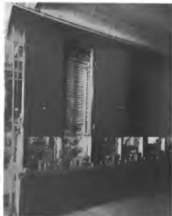
Fig. 1. Acetate Wire-Coating Machine in Operation
