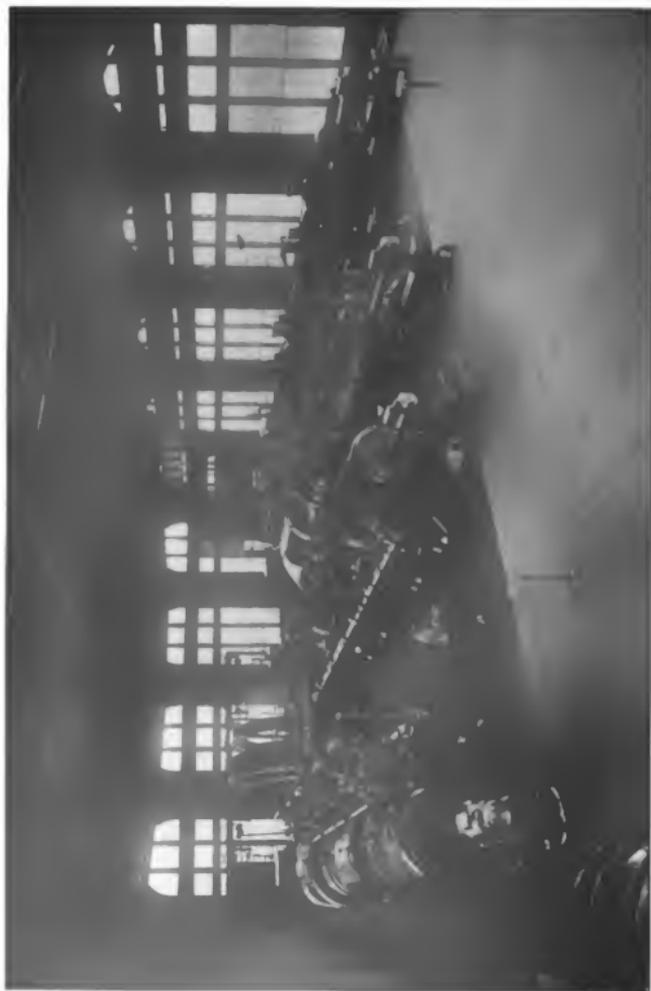
2,500 Kw. Twin Tandem Gas Engines, California Gas & Electric Co., San Francisco, Cal.
