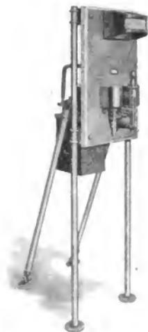
Fig. 4. Alternating Current Motor Panel on Pipe
