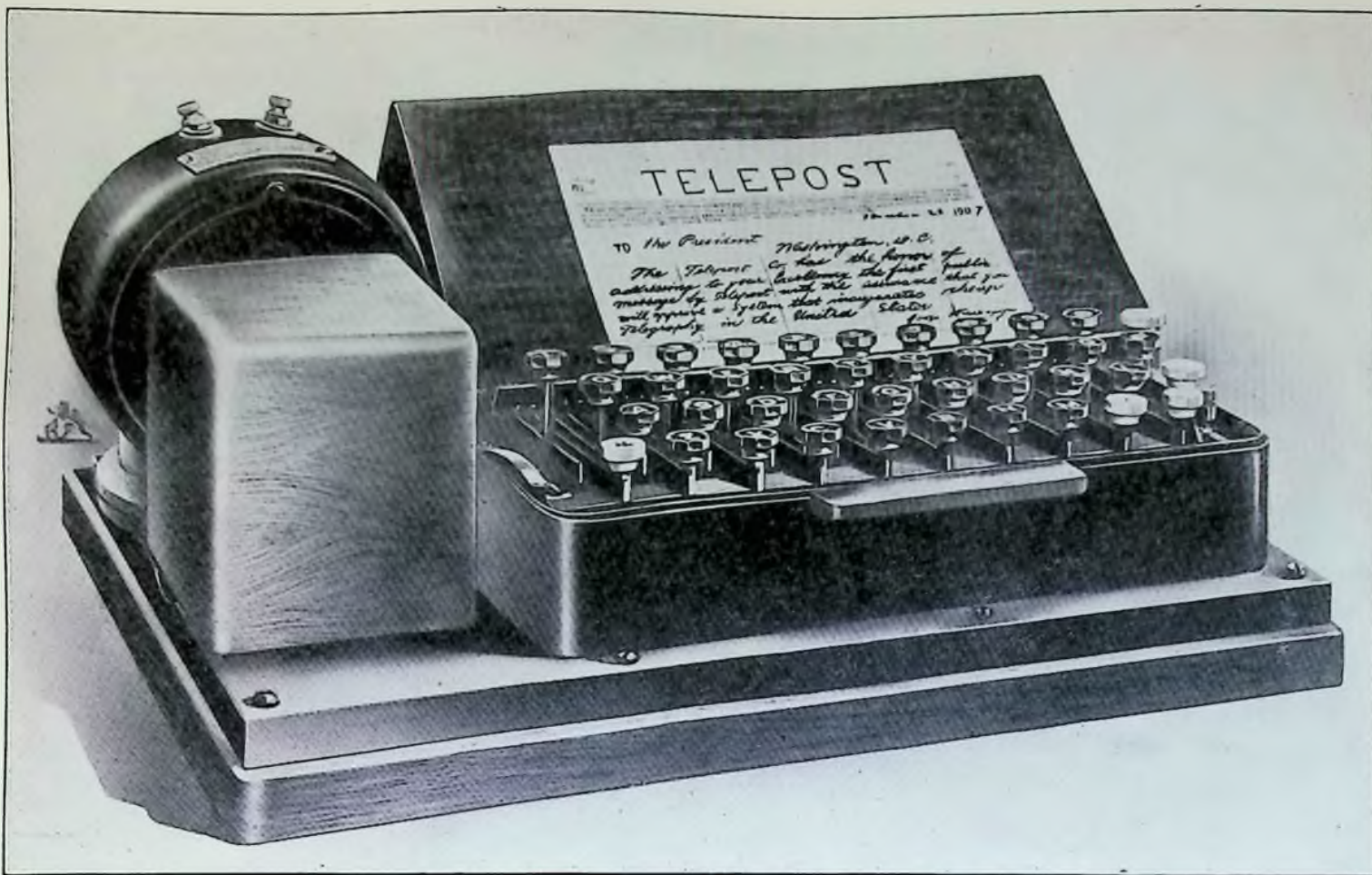
TELEPOST AUTOMATIC PRINTING TELEGRAPH SENDING DEVICE Showing First Public Message by "Telepost."
