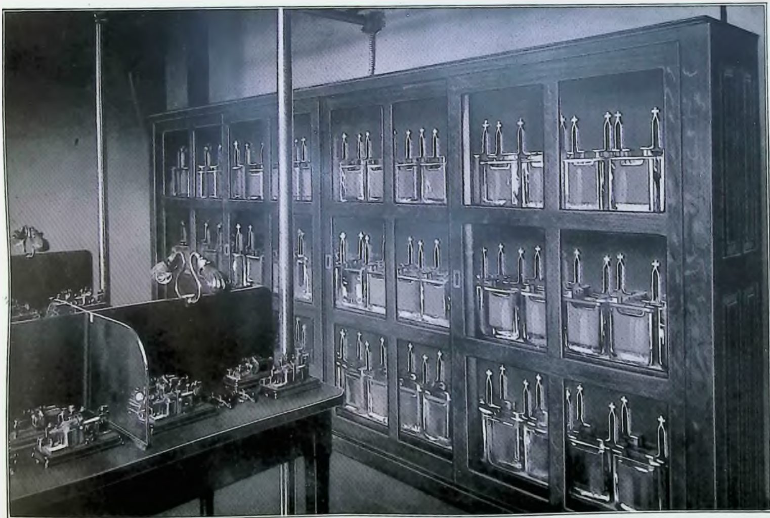
STORAGE BATTERIES AND SECTION OF TELEGRAPH TABLE U. S. Telephone Company, Cleveland, Ohio. The Dean Electric Co
