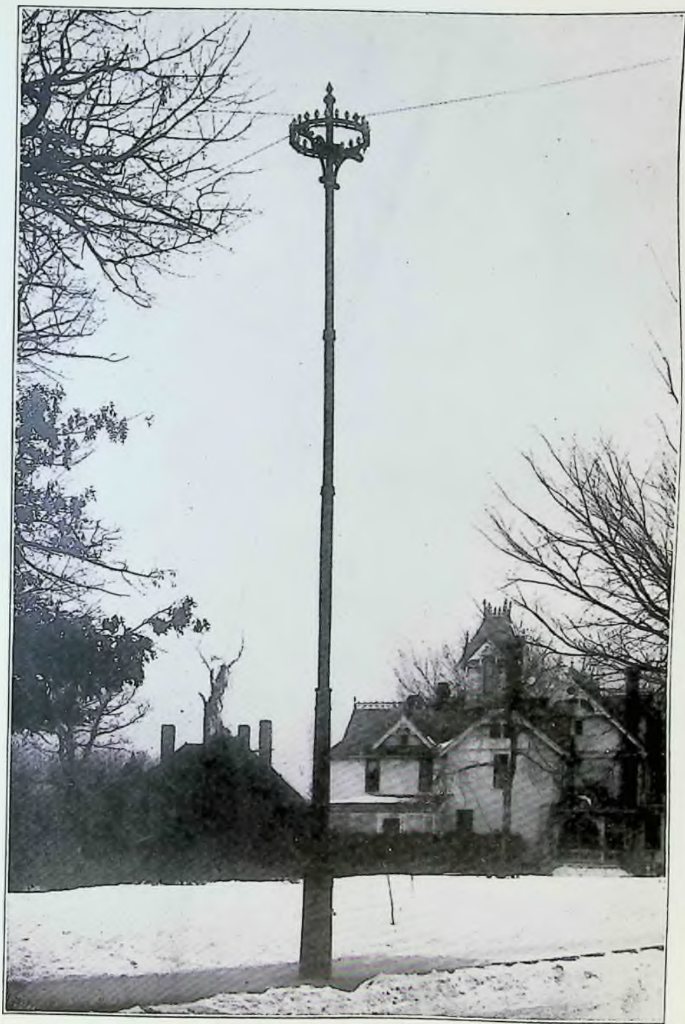
IRON DISTRIBUTING POLE Twin-City Telephone Co., Minneapolis, Minn.
