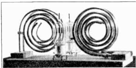
Figure 38—Spiral-Rod Oscillator.
