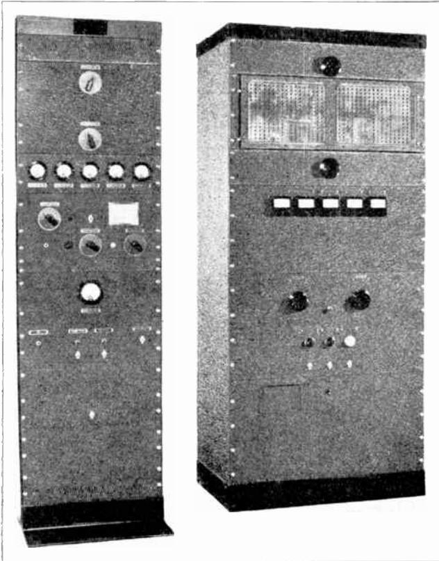
**Figure 16—The 250 watt complete radiophone transmitter (left) and high power amplifier and modulator (right).**
