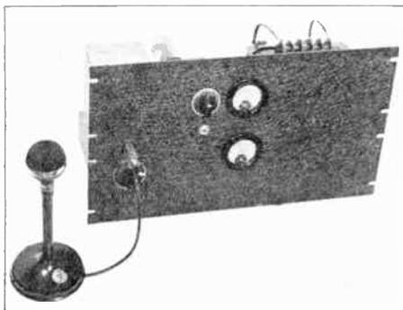
**Figure 15—Front panel view of the speech amplifier and modulator unit.**
