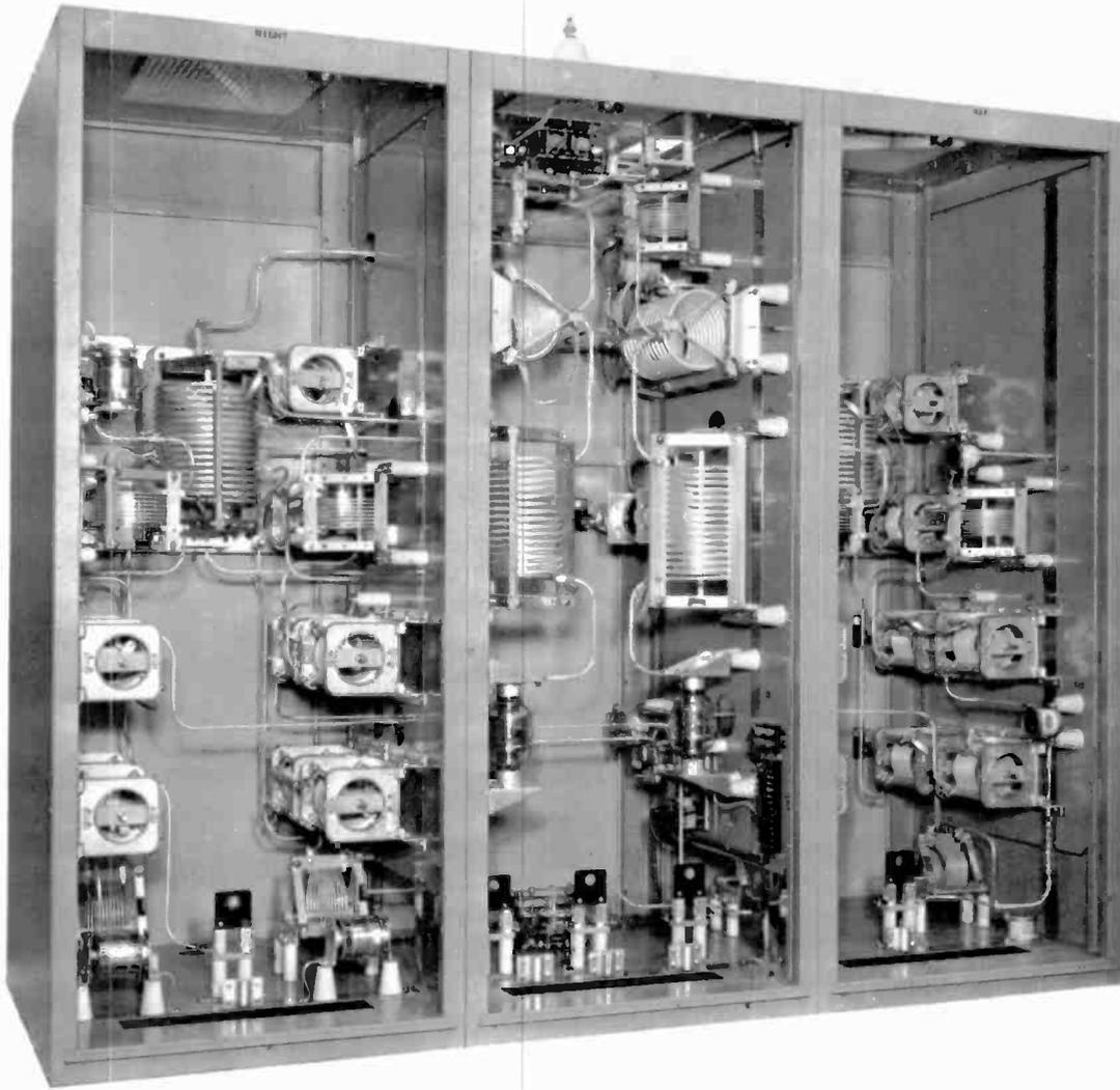
*Fig. 7-11. Phasing equipment such as this is required for a directional antenna system.*
