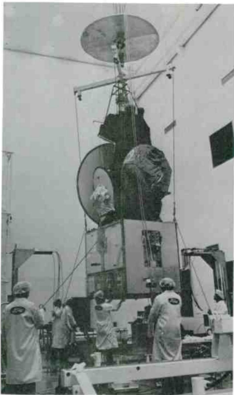
Fig. 1-10. Intelsat V being readied for launch. The satellite can handle 12,000 two-way telephone calls and two color television channels at the same time (courtesy NASA).
