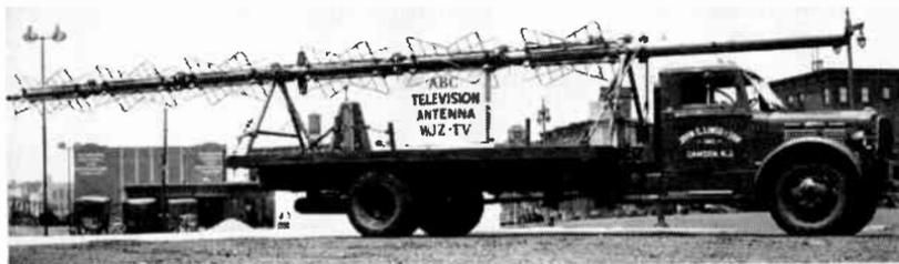
Fig. 13-38. A six-bay superturnstile antenna before erection.
