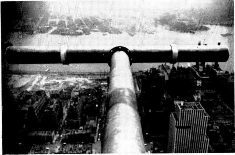
Fig. 13-35. A large-diameter broadband dipole formerly used by WCBS-TV. (Courtesy of Columbia Broadcasting System.)
