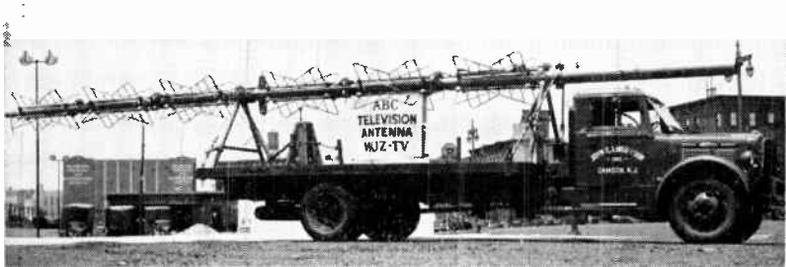
Fig. 13-38. A six-bay superturnstile antenna before erection. (Courtesy of American Broadcasting Company.)
