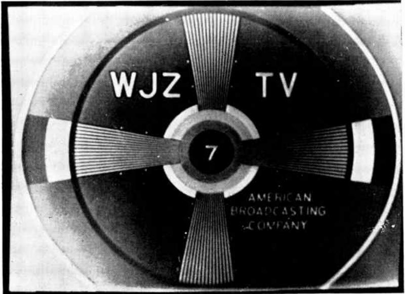
Fig. 6-19. A televised image showing the effect of iconoscope dark spot. (Courtesy of American Broadcasting Company.)
