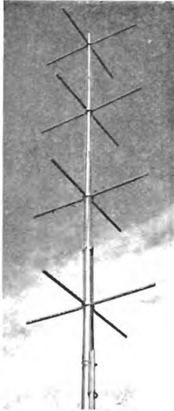
FIG. 6.26.—Close-up of an R.C.A. turnstile aerial.
