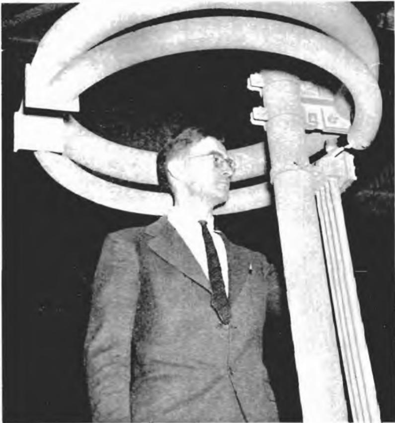
FIG. 6.32.—A close-up view of one bay of the General Electric Co., U.S.A., circular aerial, with its designer, M. W. Scheldorf.
