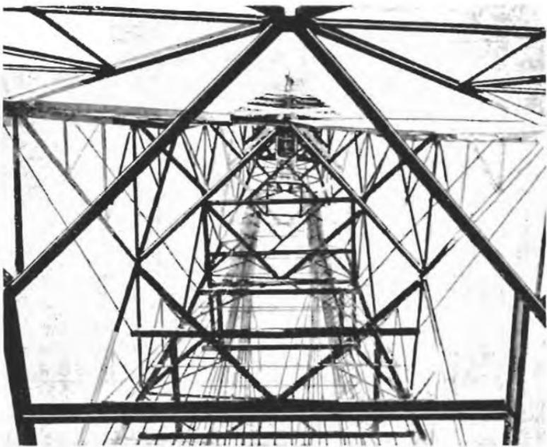
FIG. 6.29.—The co-axial cables coming down the aerial tower from the 10-bay De Mars turnstile at the 50 kW. Yankee Network F.M. station at Paxton.
