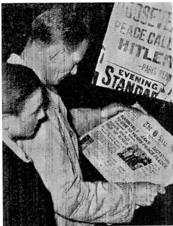
FIG. 11.3.—A commercial radiophoto picture transmitted from London to New York by the CFVD method.
