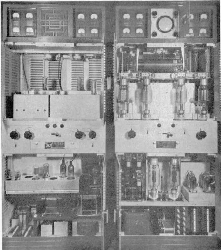
FIG. 168b.—Front of RCA 1-kw broadcast transmitter with front panels removed.
