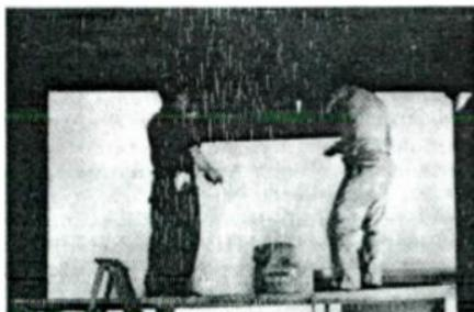
**Figure 6-1. Dielectric Welding Department in an Industrial Plant Electrostatically Shielded with Two-ounce Anaconda "Electro-Sheet" Foil Bonded to Building Paper (The shielding was applied with adhesive and the seams clinch locked.)**
