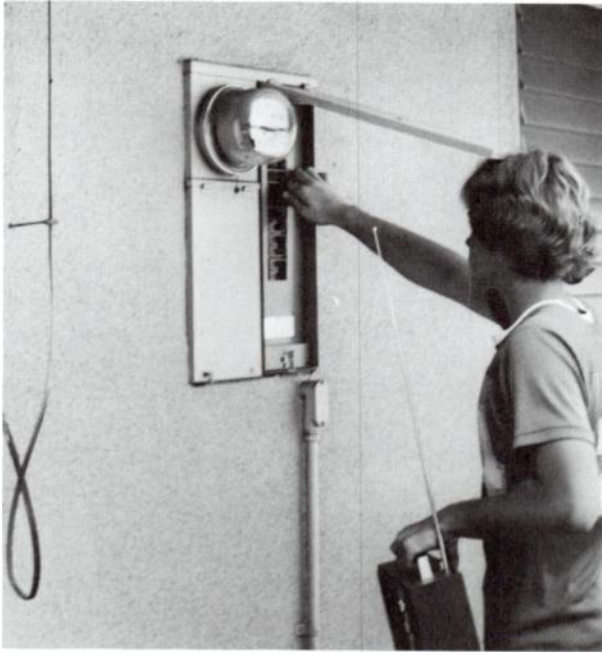
Fig. 7 With occupant's permission the electrical circuits in the residence are opened one at a time by flipping the circuit breakers or unscrewing the fuses. When the circuit serving the noisy device is opened, the interference will stop.
