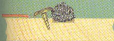
*The screw is at a slight angle so as to grip both coke and lead securely*
