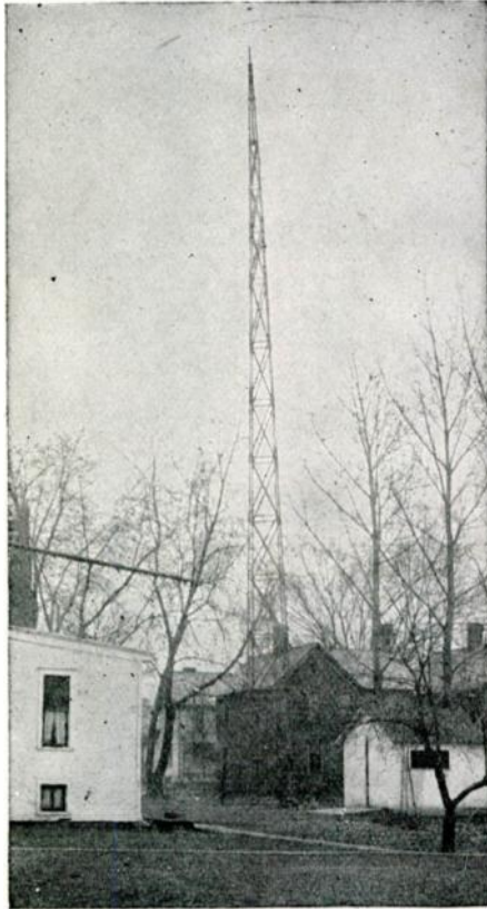
Vertical harp antenna and counterpoise of 8ZG station
