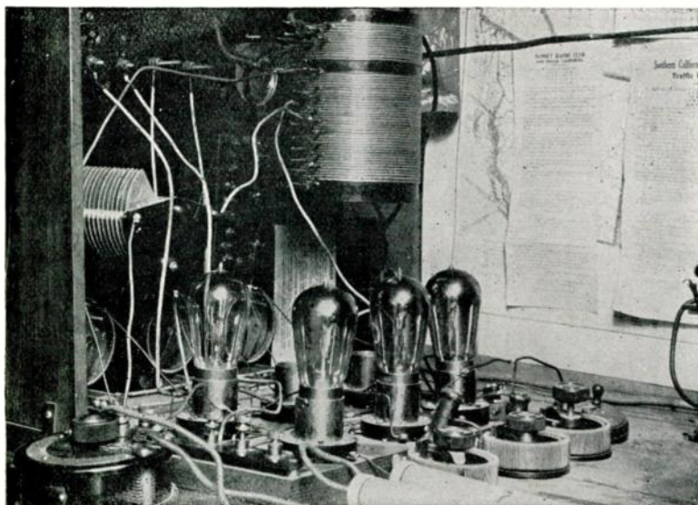
Four 5-watt tube transmitter at 6XAD with which the exceptional distance work was done
