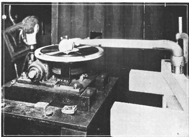
FIG. 87.—A dummy's head acting as a subject for making a test phonovision record, this latter process being visible in the foreground.
