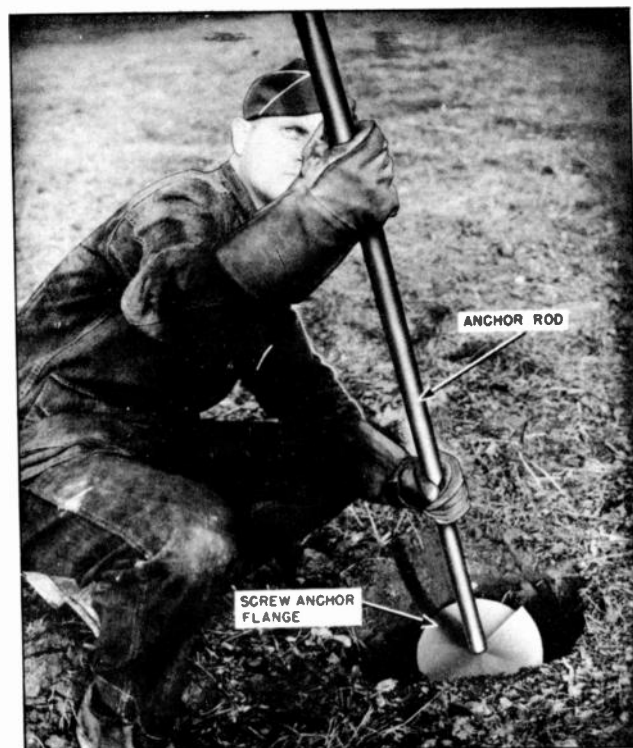
Preparing Screw-Type Anchor for Installation.
