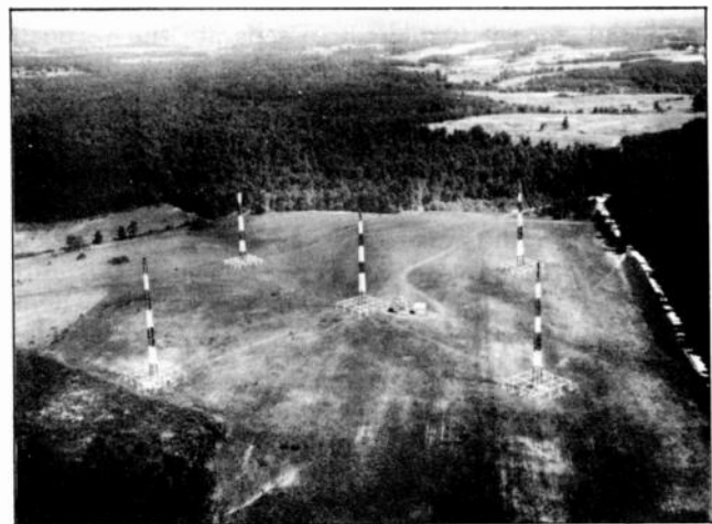
Typical Radio-Range Installation, Showing Tower Locations and Counterpoises.
