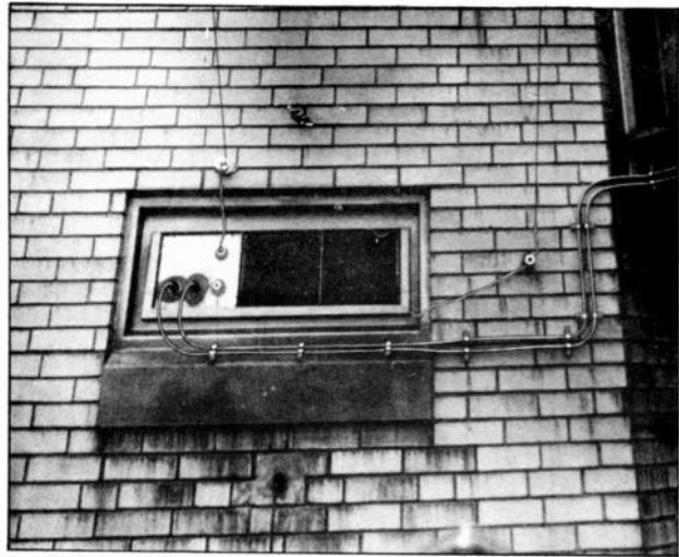
Coaxial-Transmission-Line Channelling on Outside and at Entrance to Transmitter Building.
