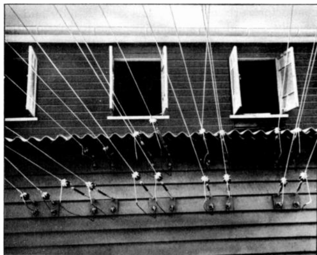
Two-Wire Feed Lines Terminated at Transmitter Building with Spring-Supported Strain Insulators.
