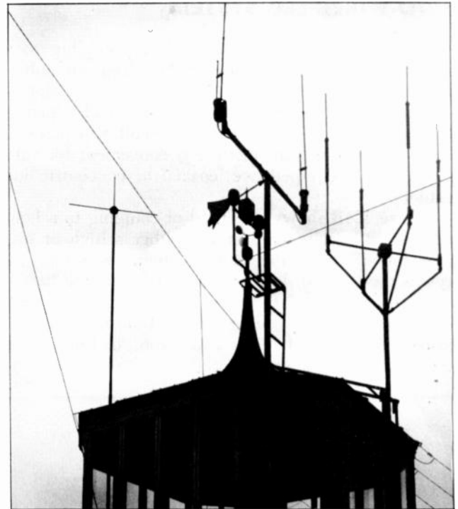
V-H-F Communication Antennas Atop a Navy-Airfield Control Tower.
