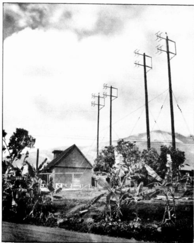
Combinations of Horizontally Polarized Stacked Dipoles and Reflectors for Directive V-H-F Radio-Telephone-Line Operation.
