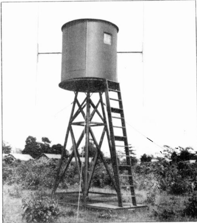
Radio-Direction-Finder Array Mounted on a Rotatable Structure.
