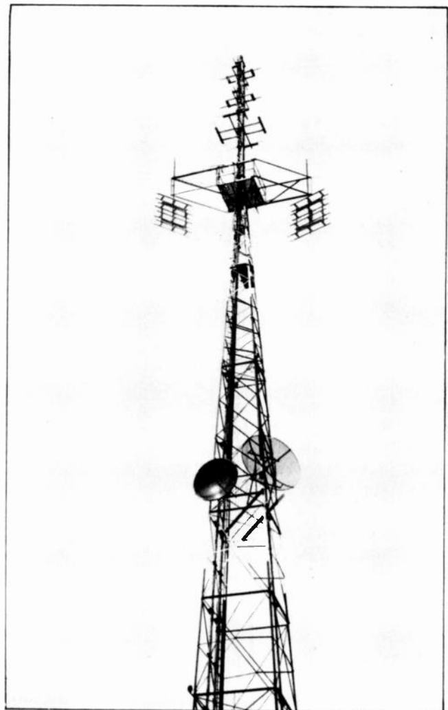
Commercial Television Tower, Showing Turnstile, Broadside, and Microwave-Parabolic-Type Antennas.
