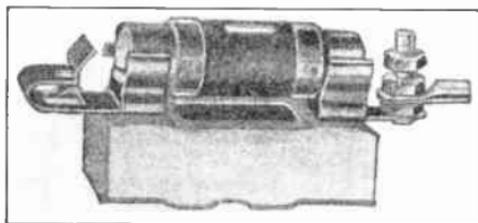
FIG. 118.—Brach lightning arrester (type 200).
