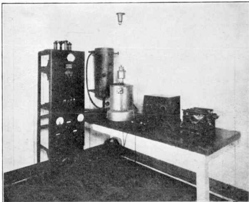
FIG. 155b.—Two-kw. Federal Arc transmitter.
