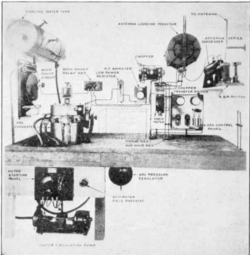
FIG. 152.—Complete arc installation.
