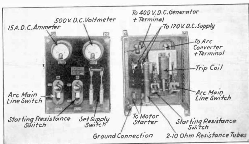
FIG. 145.—Arc-control panel.
