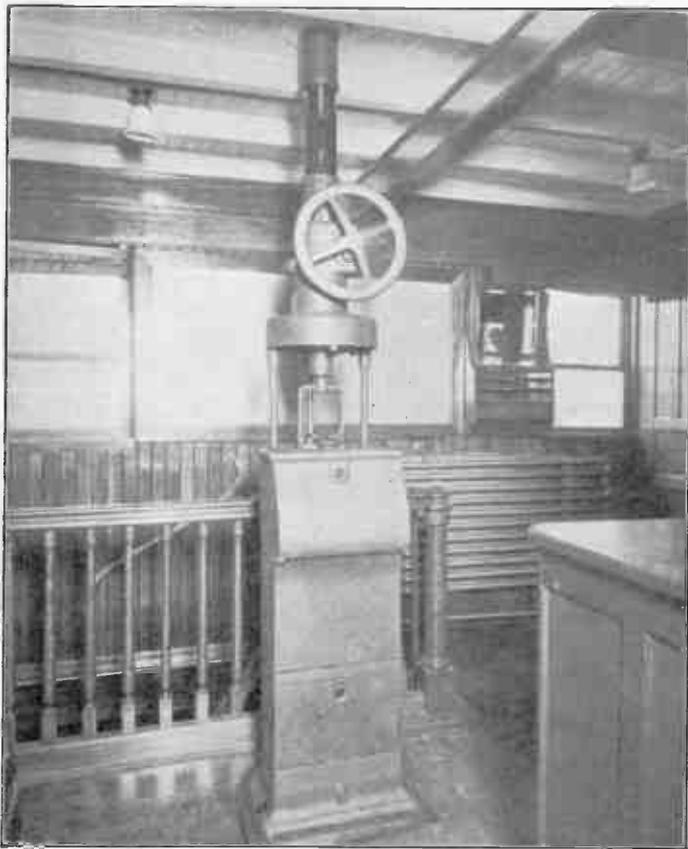
FIG. 215.—Chart-house installation of R.C.A. radio compass.
