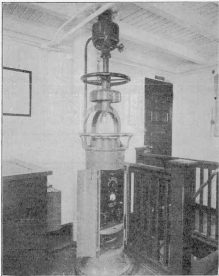
FIG. 220.—Kolster radio compass, showing panel arrangement, type AM3800.
