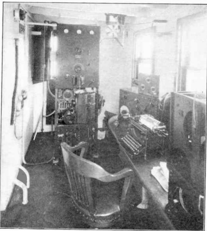
FIG. 158.—Typical shipboard installation, independent arc. S. S. Robert E. Lee.
