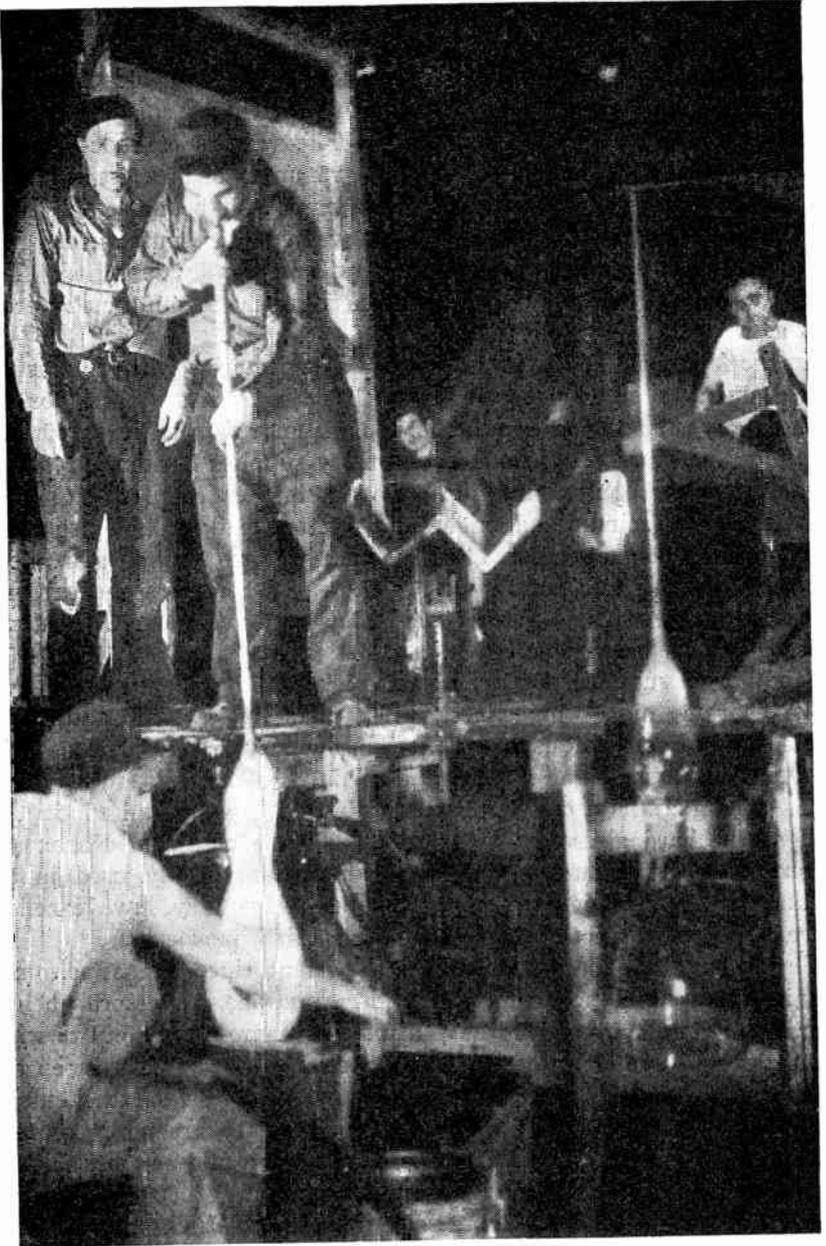
FIG. 2.36 Production of the glass blank for the cathode-ray tube at the great glass works at Corning, N.Y. To the left one sees the hot molten mass ready to enter the steel mold. To the right is the glass blank as it comes from the mold. (Courtesy of Allen B. Du Mont Labs., Inc.)
