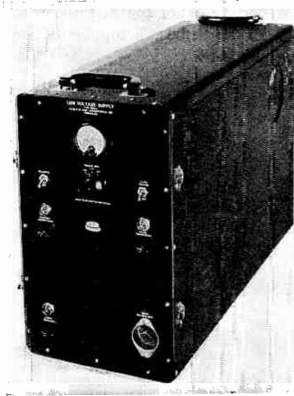
FIG. 9.18 Du Mont type 5029-A low-voltage power supply. (Courtesy of Allen B. Du Mont Labs., Inc.)
