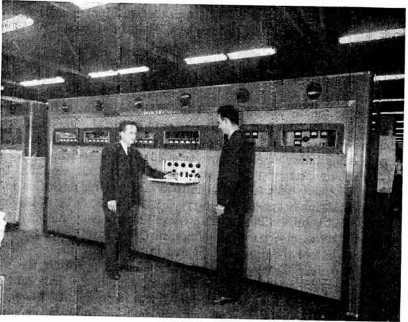
FIG. 10.15A General Electric 5-kw. Low-channel television transmitter, type TT-6-C. (Courtesy of General Electric Company.)
