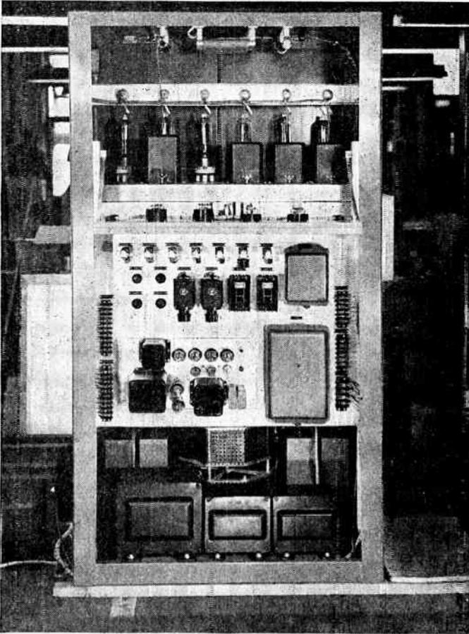
FIG. 10.9 The high voltage power supply for the power amplifier of the Du Mont master series transmitter. Covers have been removed. (Courtesy of Allen B. Du Mont Labs., Inc.)
