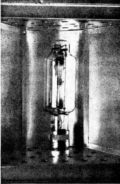
FIG. 1.2 Westinghouse type AH-12 1,000-w. mercury vapor lamp mounted in a Capital Stage Lighting Company olivette to provide a highly efficient light source at television Station WTTG, Washington, D.C. (Courtesy of Du Mont Television Network.)
