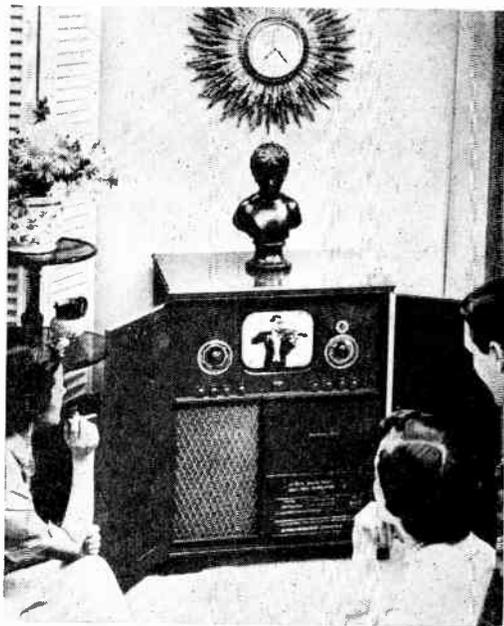
Fig. 8.4 The Du Mont Savoy receiver. This teleset is an excellent example of post-war television-receiver design. It incorporates a 12-in. picture tube, includes an automatic record changer, and provides continuous tuning throughout both the FM and TV bands. An AM receiver is included. (Courtesy of Allen B. Du Mont Labs., Inc.)
