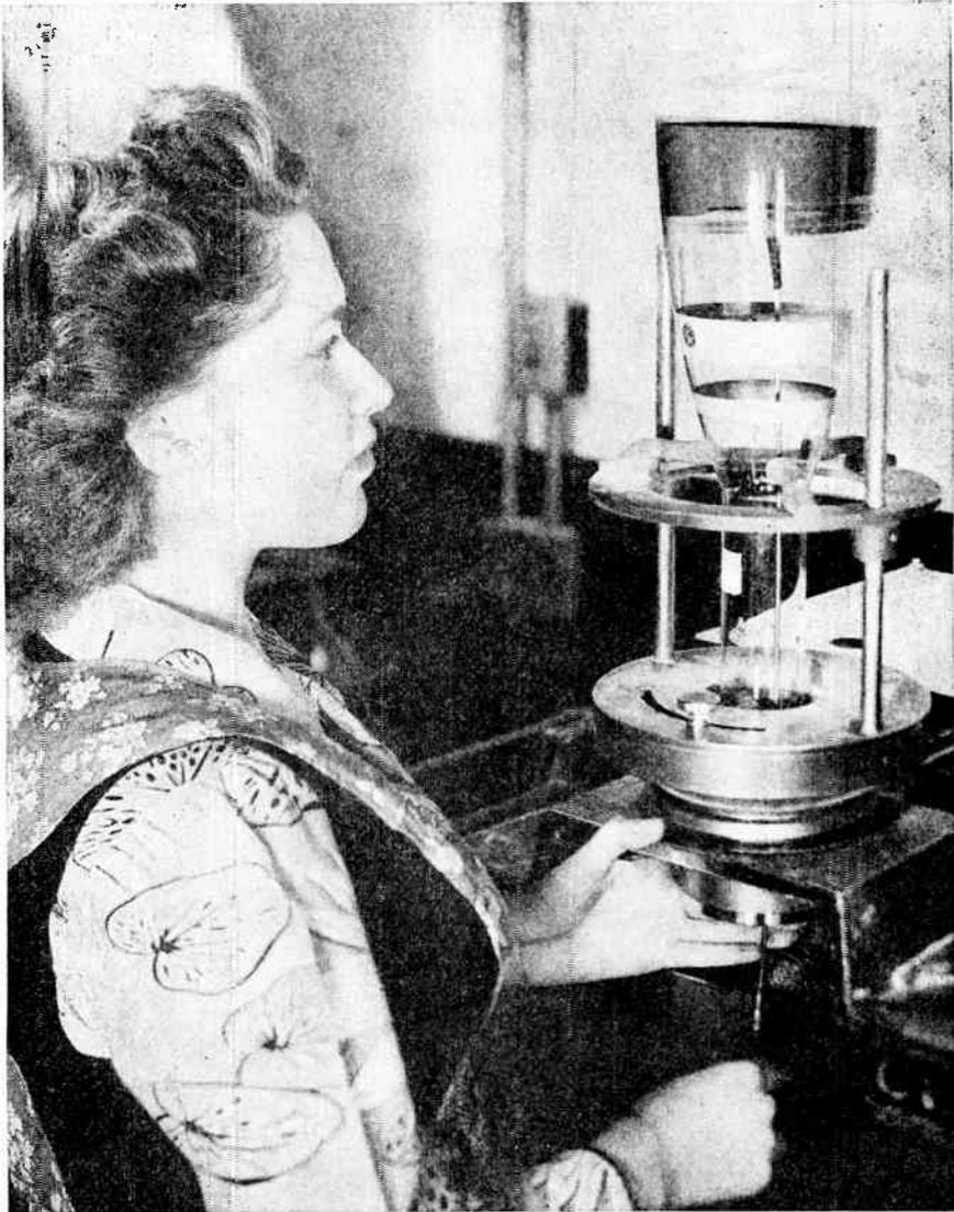
FIG. 2.14 Method of applying a coating of electrically conductive material to a cathode-ray tube, creating an electrode upon the interior walls of the tube, which serves to accelerate the beam as well as to remove electrical charges from the walls of the tube. (Courtesy of Allen B. Du Mont Labs., Inc.)
