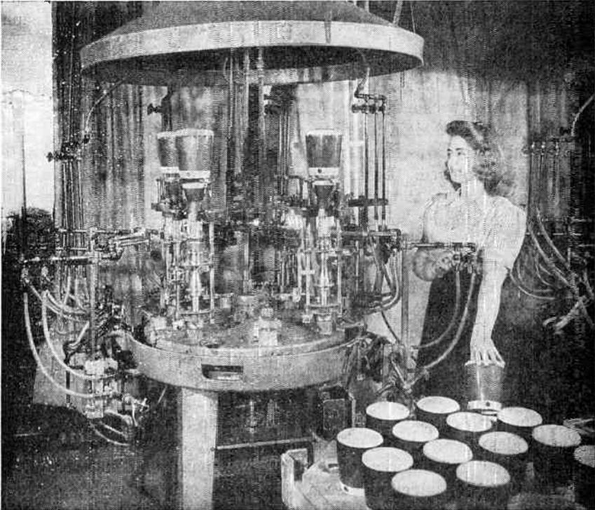
FIG. 2.37 Complete gun and stem assembly being sealed to the already-prepared blank on an automatic sealing machine. (Courtesy of Allen B. Du Mont Labs., Inc.)
