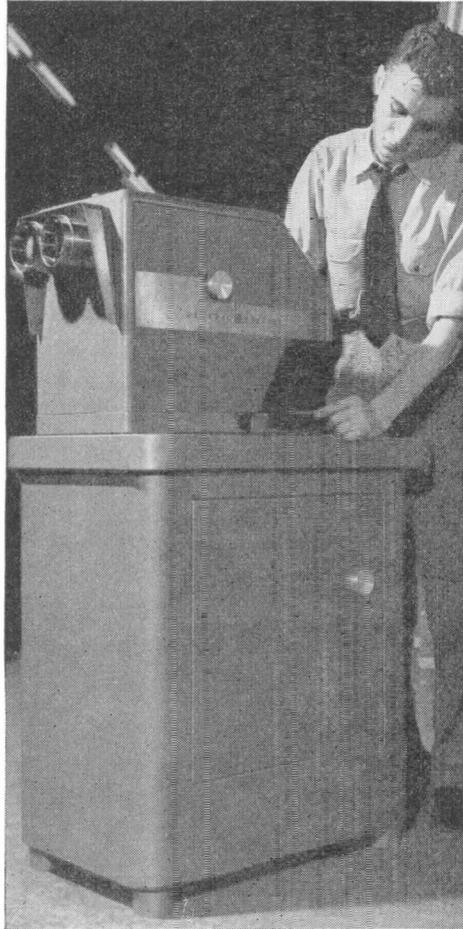
FIG. 11.34 A General Electric slide projector, type PF-3-C for television. This dual projector will accommodate standard slide transparencies, switching of slides being accomplished at the projector proper. With the dual-projector arrangement, one slide may be televised while the slide holder of the second projector is being loaded. Thus, rapid switching of slides may be accomplished. (Courtesy of General Electric Company.)
