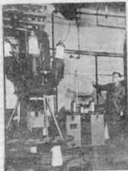
FIG. 1 (above).—A 500 kW, 12,500-VOLT HIGH VOLTAGE SEALED STEEL TANK RECTIFIER ENCLOSURE IN A TRANSMITTING STATION.
