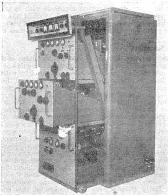
FIG. 18.—A MEDIUM-POWER TRANSMITTER, GIVING 750 WATTS ON C.W. AND 500 WATTS CARRIER ON M.C.W. OR TELEPHONY, IN THE BANDS 137-650 kc/s OR 2-25 Mc/s.
