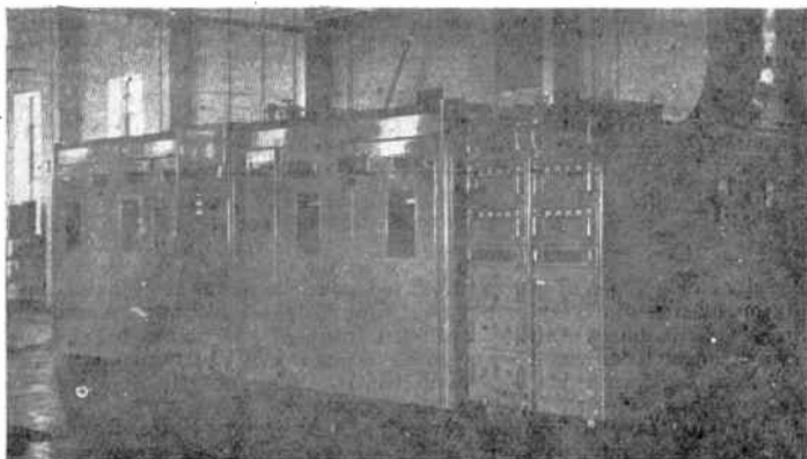
FIG. 24.—D.S.13. 40-kW PEAK POWER TRANSMITTER AND A1406/A1407 I.S.B. DRIVE AND MONITORING EQUIPMENT.
