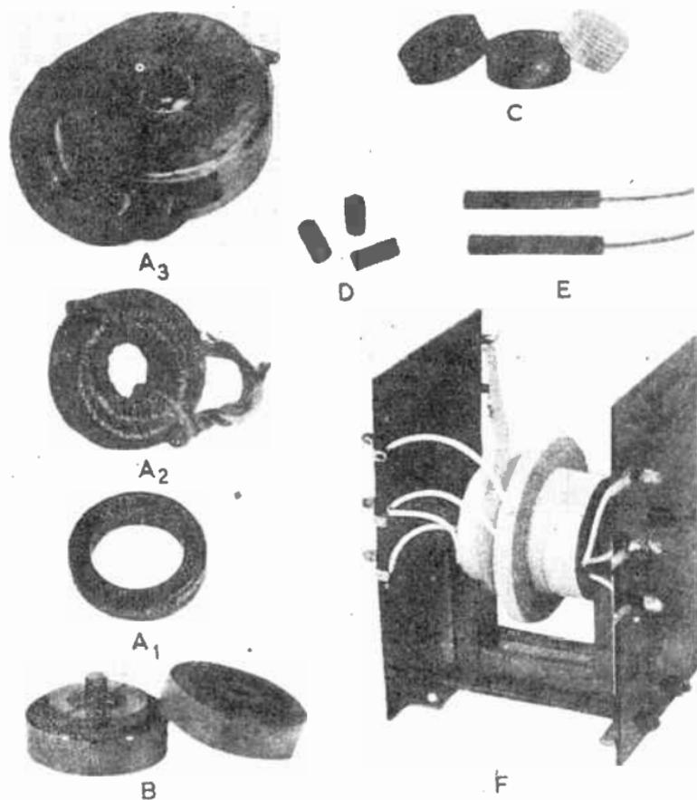
FIG. 4.—VARIOUS TYPES OF MAGNETIC POWDER CORES.
