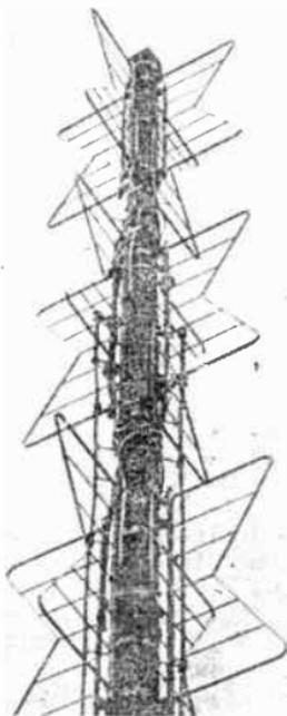
FIG. 25.—THREE-STACK SUPER-TURNSTILE TELEVISION AERIAL.
