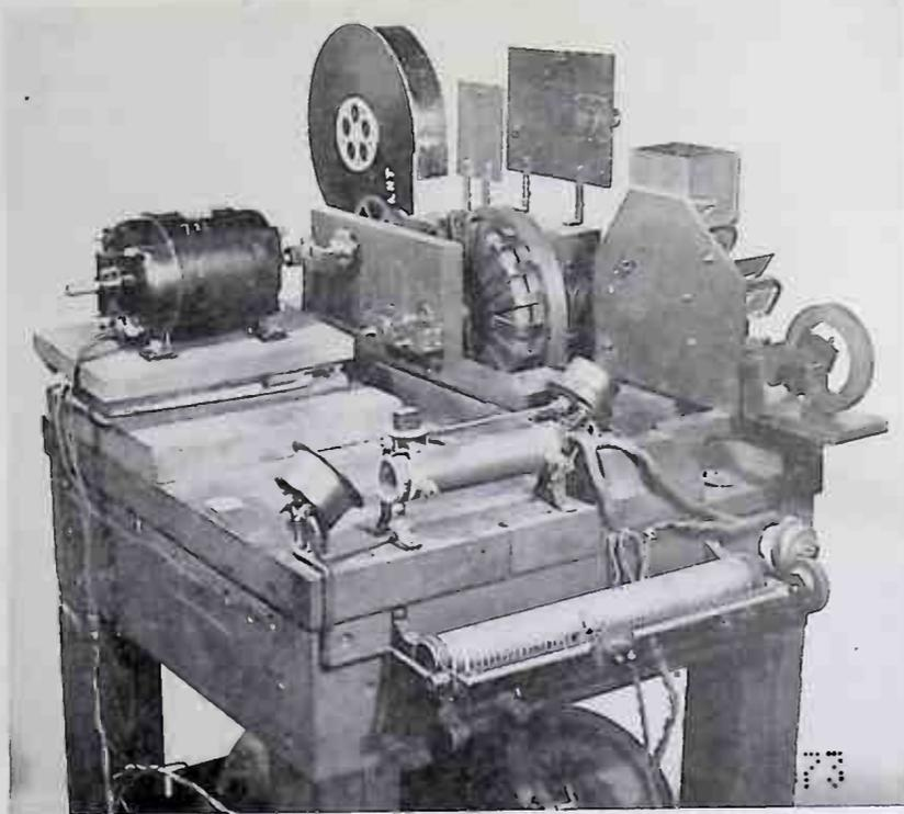
Fig. 6. Original model of magnetic-drive recorder.
