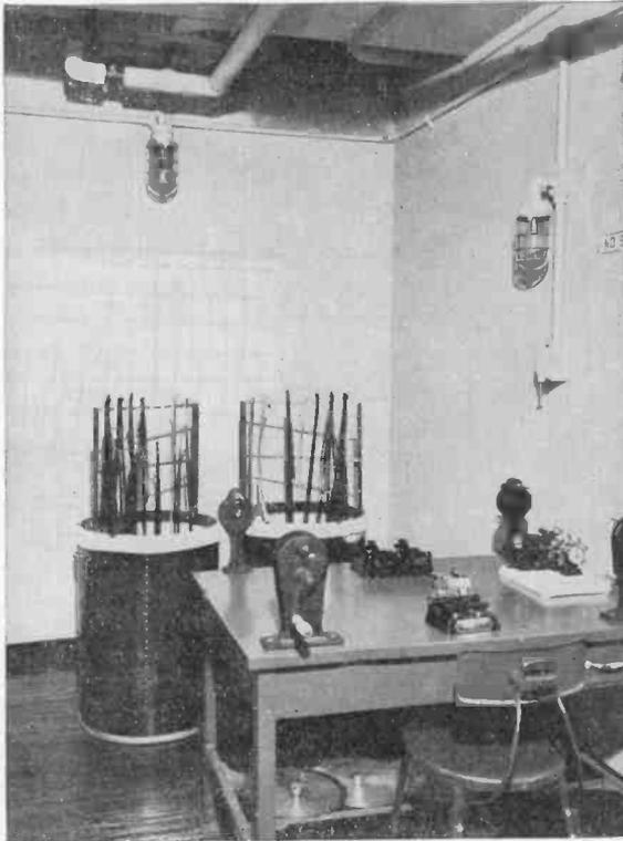
FIG. 14-5. A neatly arranged rewind room containing the various accessories required for efficient film-handling operations. Note the explosionproof lighting fixtures and switches, the fireproof construction of all furniture and fittings, and the water sprinkler system. (Courtesy of WCAU-TV, Philadelphia.)
