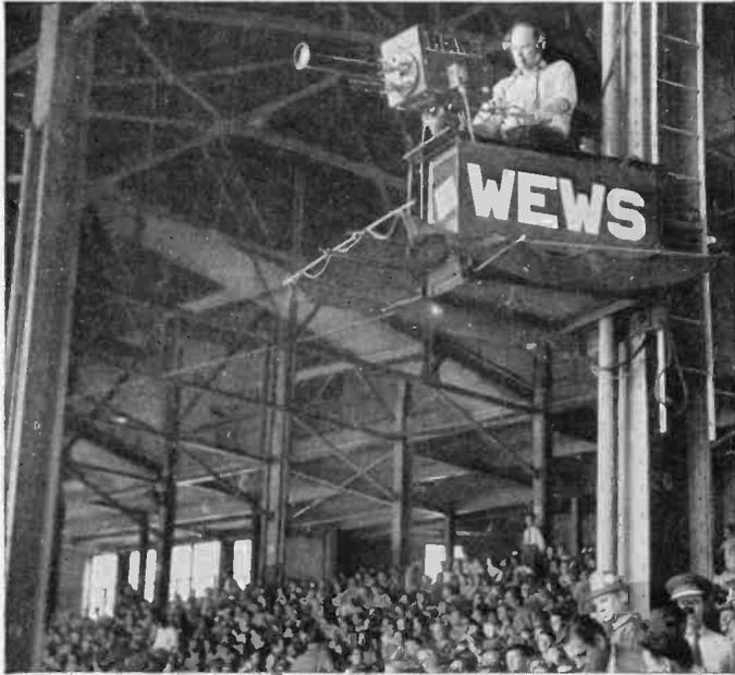
FIG. 4-4. This especially constructed camera platform, on one face of a steel column, provides a camera position at a vantage point that otherwise would not have been available. The crow's-nest appearance is created by the installation of netting to catch any objects that might be dropped accidentally. (Courtesy of WEWS, Cleveland.)
