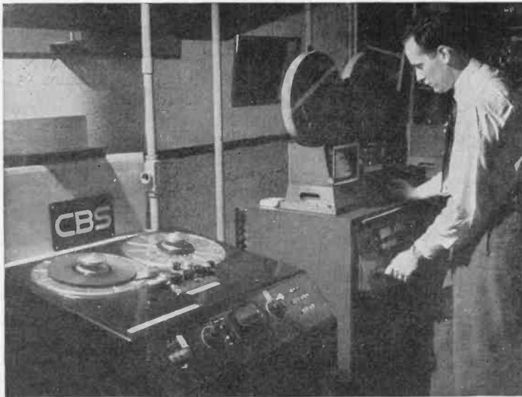
FIG. 11-2. A sound recording corner of a television recording room showing a synchronous,  $\frac{1}{4}$ -in.-wide magnetic-tape recorder at the left and a 16-mm sound-on-film recorder at the right.
