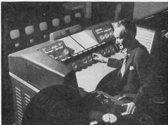
FIG. 6-21. A completely self-contained studio audio control console which contains adequate facilities to accommodate the most complex type of television production.
