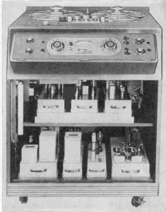
FIG. 11-17. A magnetic-tape recorder that handles  $\frac{1}{4}$ -in.-wide tape and which, with the aid of a control track, is capable of recording and reproducing sound in exact synchronism with an associated picture.
