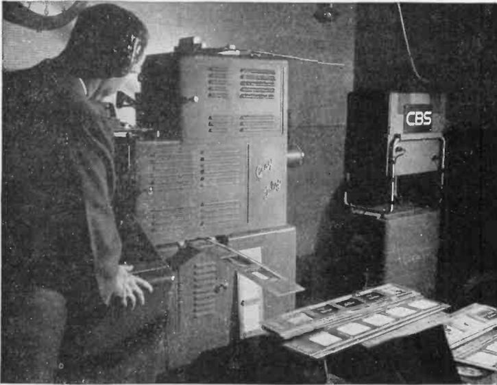
FIG. 9-4. The telop at the left is handling opaque copy in its top and bottom ports and projecting the material onto an iconoscope camera tube contained in the housing at the right.
