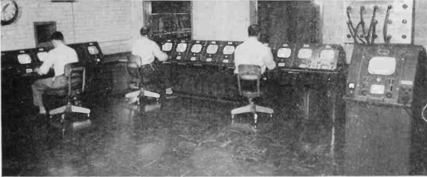
FIG. 14-23. All the camera-control units for two medium-size studios, two announce studios, and a telecine room are concentrated in this single control room which thus serves the entire studio plant. This arrangement eliminates the need for camera-control units in the individual studio control rooms. (Courtesy of WOR-TV, New York.)
