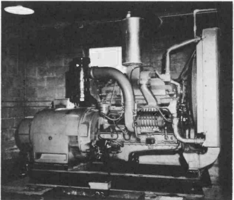
Fig. 8-16. Diesel-driven generator used to supply emergency power for the transmitter at station WTAE.
