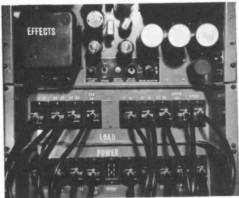
Fig. 2-17. Typical power-supply patch panel as installed at WISH-TV.
