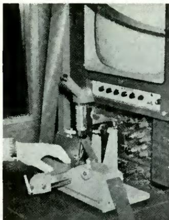
(E) Drape tape from supply reel over tape support post and position under left hold-down door.
