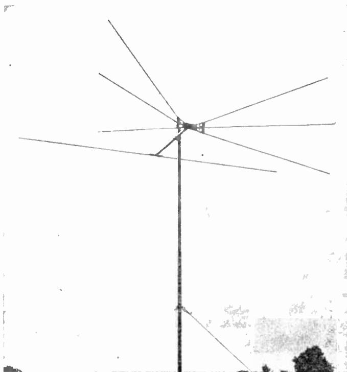
Fig. 253 Channel Master Fan Conical (Courtesy of Channel Master Corporation)
