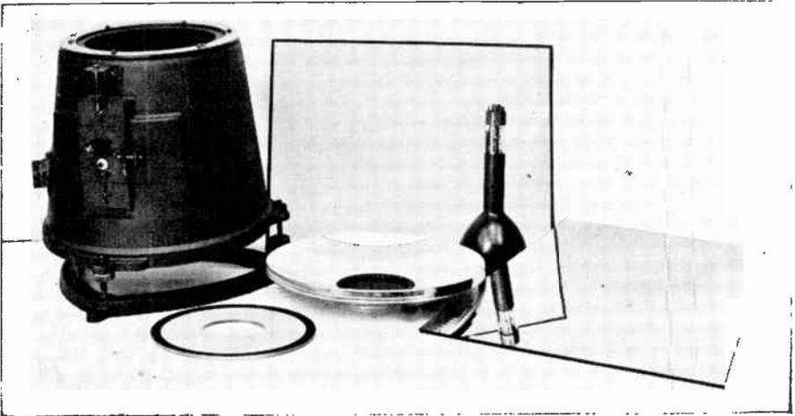
FIG. 231 Components of RCA Projection System
