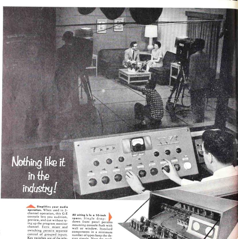
Key switches are of the telephone type. There are no push buttons anywhere!
