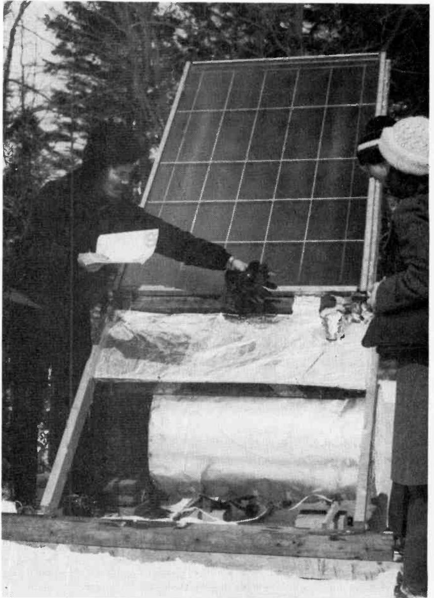
*Mark Cairenius of Markko Construction points out the details of the special low energy requiring circulation system in their solar collector design. Although this prototype is a fairly typical flat plate design, the use of black particles suspended in the liquid have resulted in very efficient heating.*
