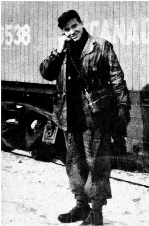
● Tests to determine if radio-telephone communication can increase the speed and efficiency of handling freight trains are being carried out by the Canadian National Railways on its fast Montreal to Vancouver freight trains. The experiments are the first of their kind undertaken in North America
