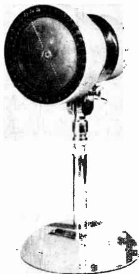
The sensitivity naturally varies with the type of aircraft transmitter used, but bearings obtained are accurate to distances as great as those at which voice communication can be maintained between the tower and the aircraft.
