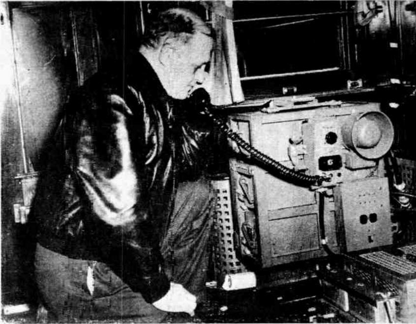
● An engineer demonstrates the use of radio-telephone communication on Canadian National Railways freight trains between Montreal and Vancouver. The tests, the first of their kind in North America, permit instant communication between head and rear end crews and wayside stations.
