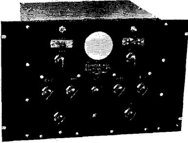
● Controlled linear sweep 0-150,000 C.P.S. ● Controlled external sweep. ● Freq. locking device for sweep frequency. ● Picture centering adjustments. ● Wide range focus adjustments. ● Complete component shielding. ● Unit is self contained and includes batteries and 110V-60 cycle power supply. ● Tubes RCA 906-385-234-281-280. ● This instrument embodies all features ordinarily contained in only the highest priced Cathode Ray equipment.
