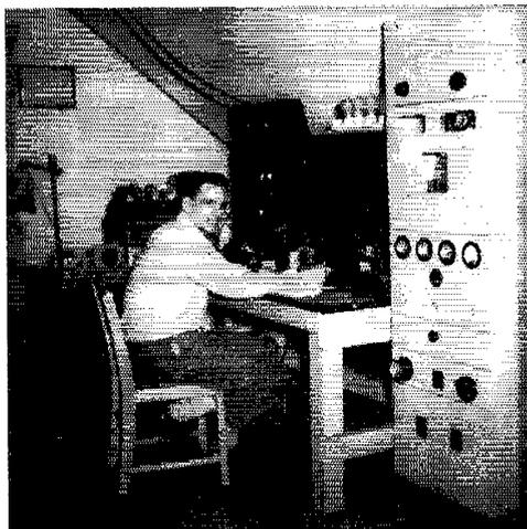
Here is Bob Ehrlich, W2NJR, of West Orange, N. J., and his neat shack and rig. The rack at the right houses the 833A final and its power supplies, while on the table the left-hand rack carries the exciter and its 807 driver-amplifier, with a BC-348 receiver in the right-hand rack. The table at the rear carries a 'scope and some 2-meter gear (not s.s.b., yet). Bob is one of the early-birds in s.s.b., and authored that excellent article on linear amplifiers in the May issue.
