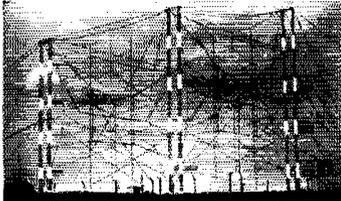
Designed, built and installed by Trylon, these two broadbands give 5% to 10% more reliable long-distance communications than comparable rhombics — and with a bandwidth of ±15% of center frequency at 1.5 VSWR.
