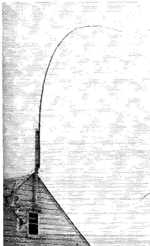
Here's what the ice did to W1VG's 40-meter ground-plane antenna during one of our better New England days. But after the sun came out the antenna returned to normal.
