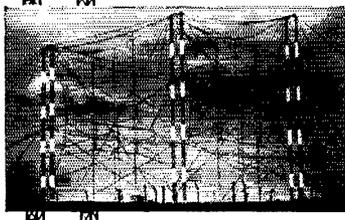
Designed, built and installed by Trylon, these two broadsides give 5% to 10% more reliable long-distance communications than comparable rhombics — and with a bandwidth of  $\pm 15\%$  of center frequency at 1.5 VSWR.
