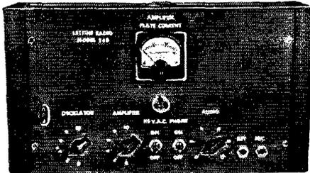
**MOD. 240 WITH MOBILE CONNECTIONS & AC SUPPLY**
