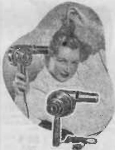
These Hair Driers are moulded in beautifully finished bakelite. They are British made, the fan being driven by a solidly constructed and trouble-free motor. A heating element is incorporated and a switch provided so that hot or cold air can be obtained at will. As a quick and efficient means of drying the hair, these electrical hair driers are ideal.
