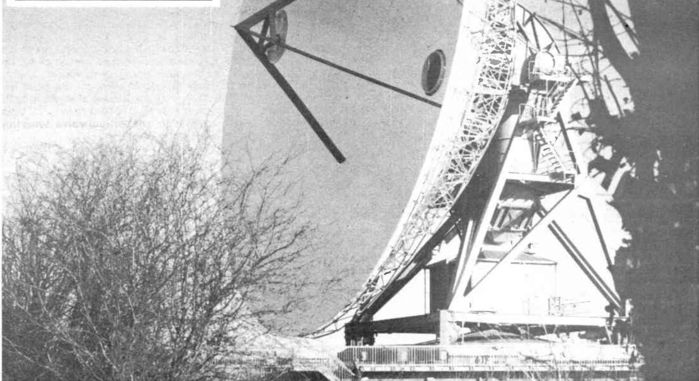
tion. This time made of aluminium, the dish measured 97 feet in diameter, and worked on the Cassegrain principle as did its predecessor. The unit moved in azimuth and elevation on bearings mounted at the top of a reinforced concrete tower six feet tall. The use of aluminium gave a further weight-reduction of the system to 331 tons.
