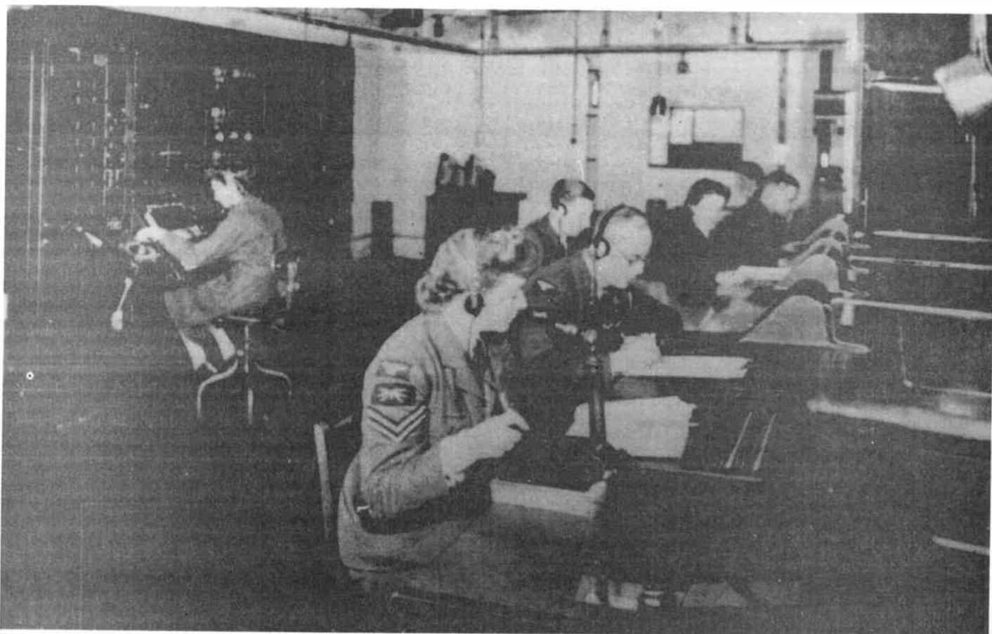
Inside the receiver room of an East Coast Chain Home station. The WAAF at the left rear can be seen operating the goniometer while observing the display tube
